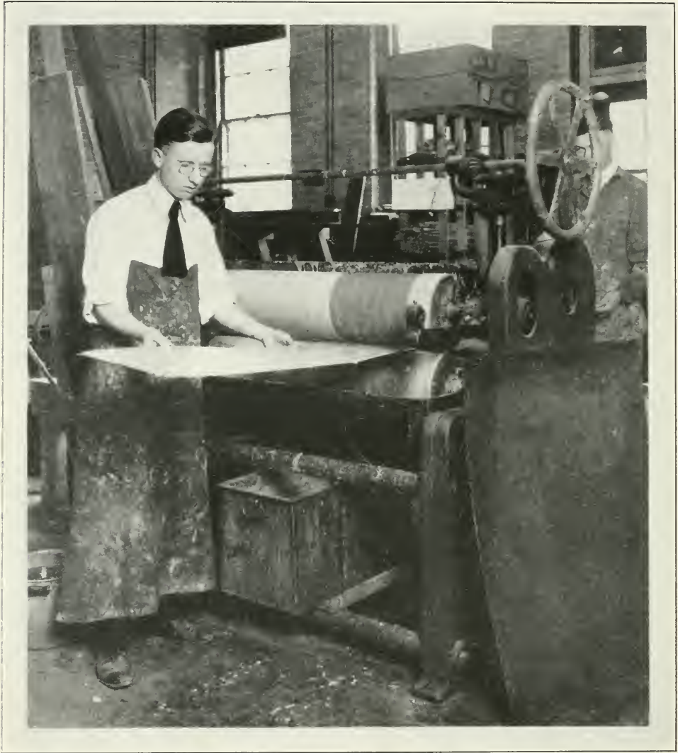
GLUE SPREADING MACHINE—A STEP IN THE MAKING OF PLYWOOD
