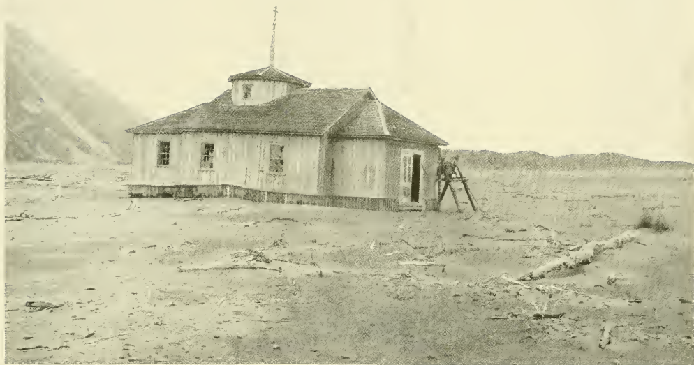
THE GREEK CHURCH AT KATMAI VILLAGE STANDING IN THE MUD AND WRECKAGE LEFT BY THE GREAT FLOOD
