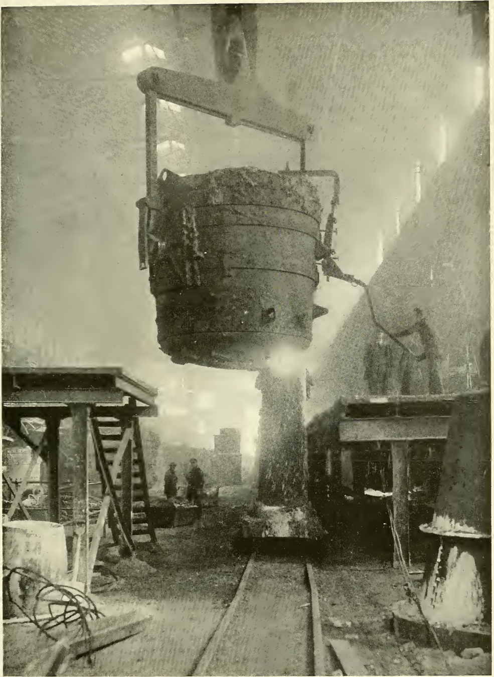
CASTING THIRTY TONS OF MOLTEN STEEL IN ONE OF CANADA'S LARGE STEEL PLANTS
