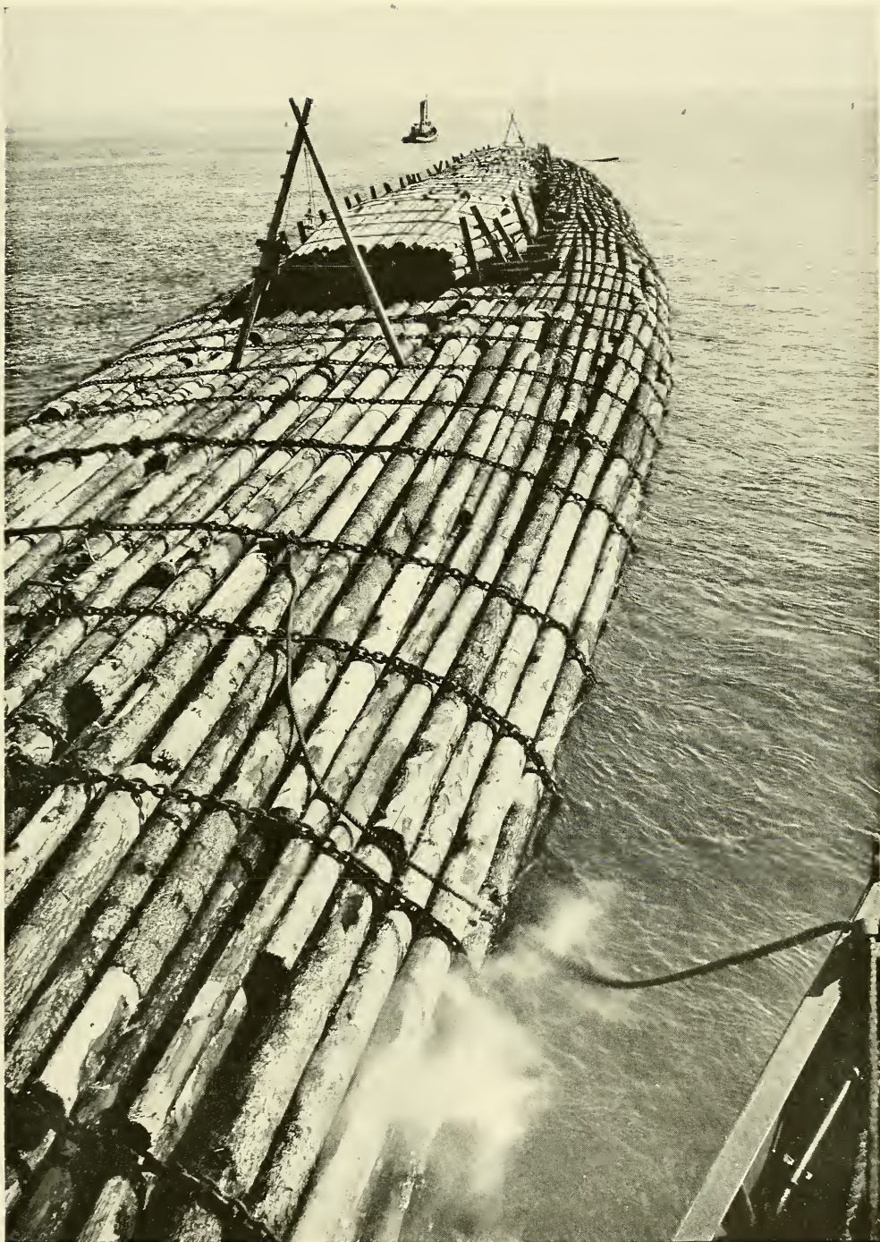
BRINGING INTO SAN DIEGO HARBOR A LOG RAFT CONTAINING 5,000,000 FEET The raft has journeyed down the coast from Portland, Oregon, where this type of raft was invented
