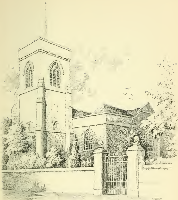
ST NICHOLAS CHURCH DEPTFORD East Street
