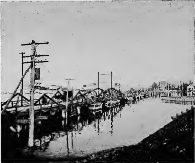
OLD CITY ISLAND BRIDGE
