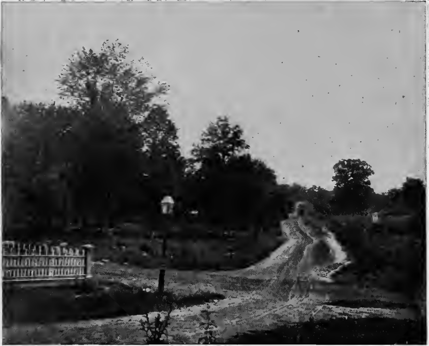
HOME STREET, LOOKING EAST FROM UNION AVENUE IN 1883
