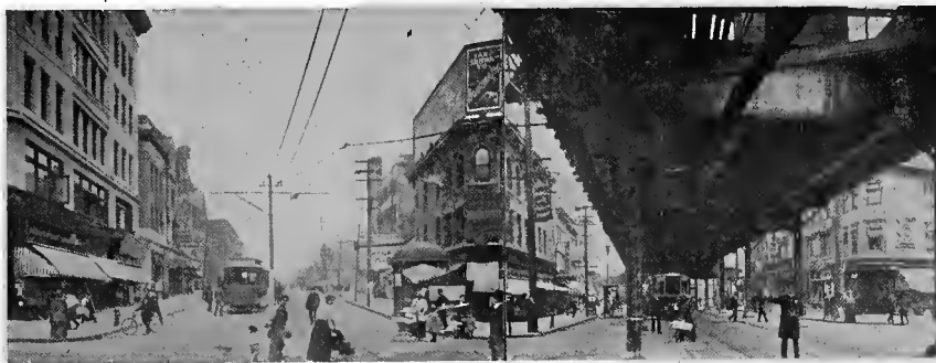
JUNCTION 149TH STREET AND THIRD AVENUE
