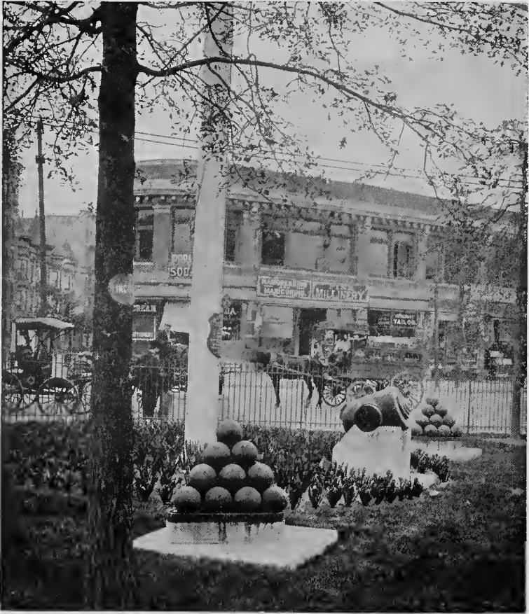
MCKINLEY SQUARE—169TH STREET AND BOSTON ROAD
