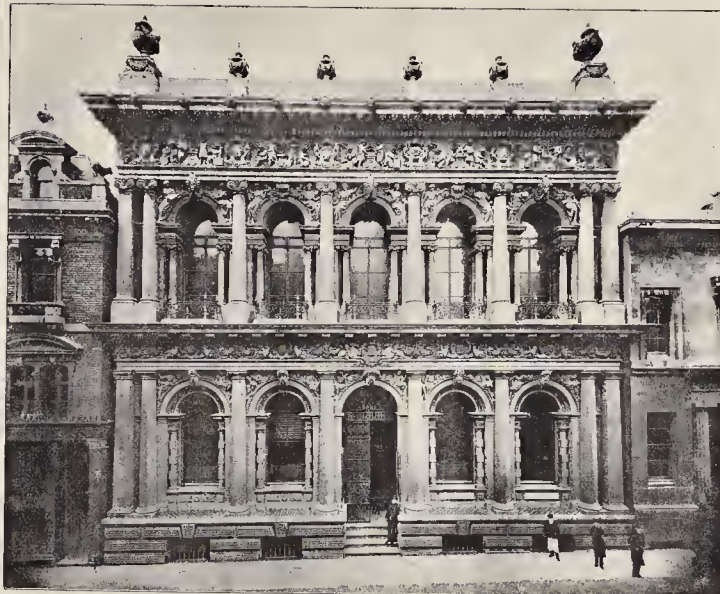
LLOYDS' BANK BUILDINGS.
