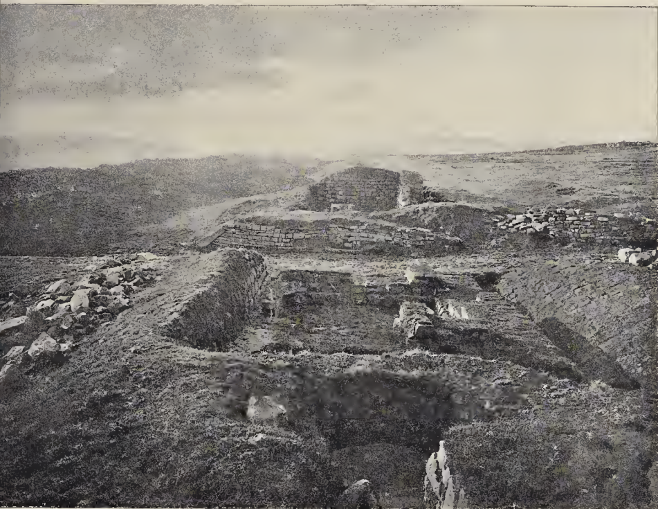
SOUTH GATEWAY, ÆSICA; FROM EAST.
