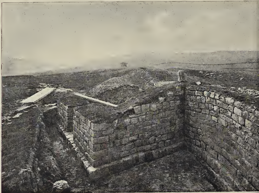
NORTH-WEST ANGLE TOWER, ESICA.
