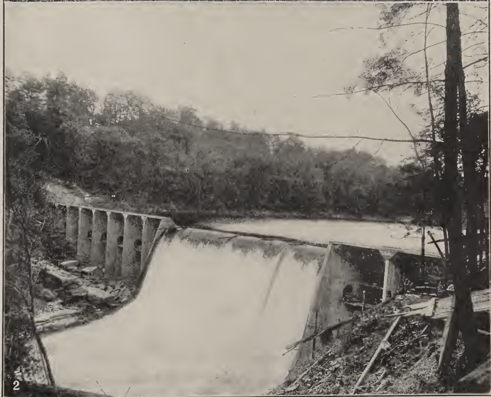
1. A REINFORCED-CONCRETE GRAIN ELEVATOR AT CHICAGO, ILLINOIS 2. A REINFORCED-CONCRETE HOLLOW DAM AT CUYAHOGA FALLS, OHIO
