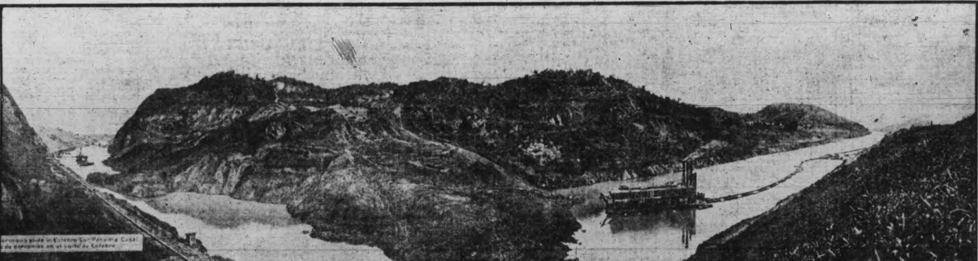
This slide which occurred several weeks ago in the Culebra Cut of the canal is holding up a large amount of shipping, and huge efforts are being put forward to clear the passage once again. It is believed, however, that not until December will ships find it possible to get through the canal.
