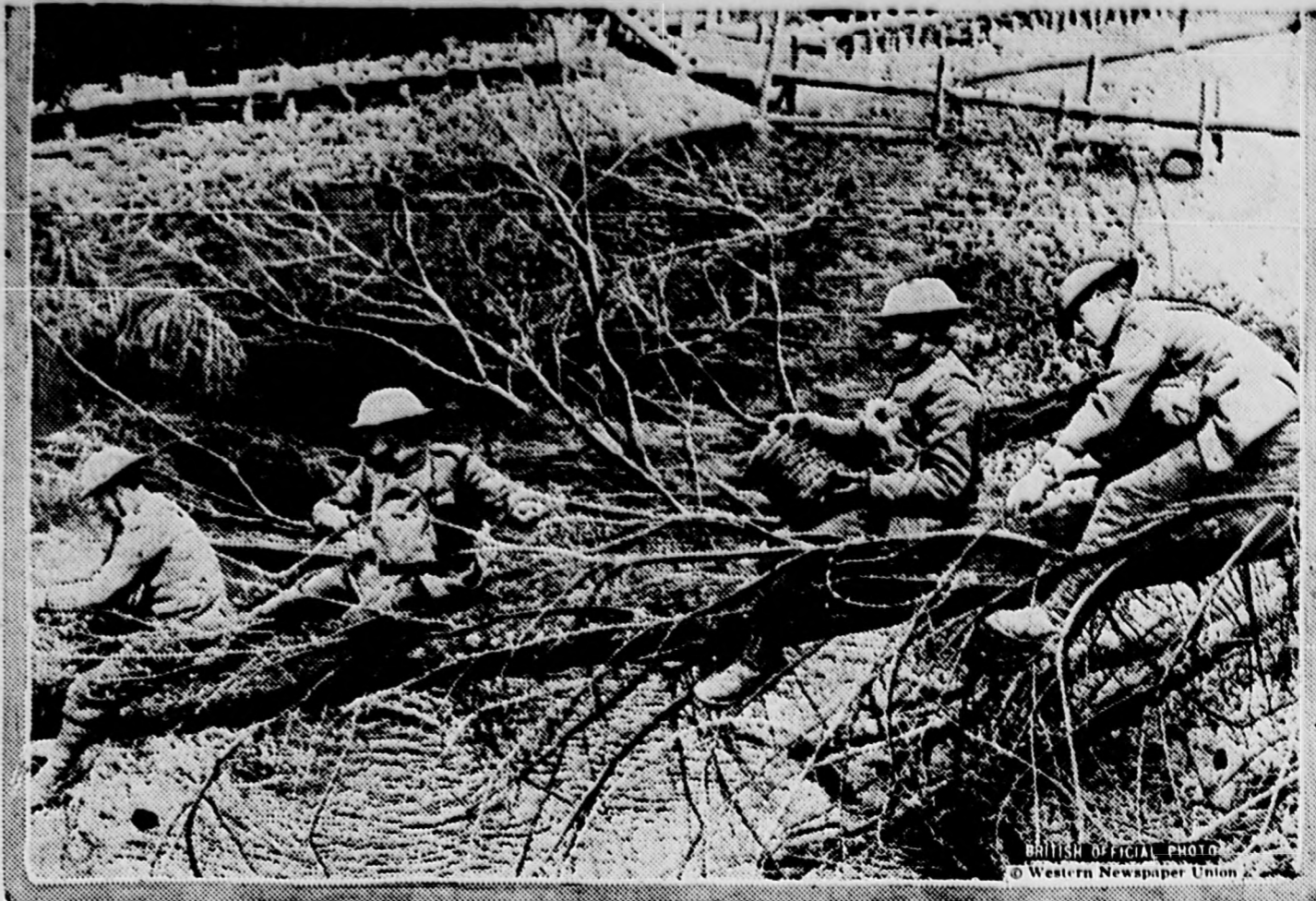
British wiring trees which they have felled across a canal to hold up the enemy.
