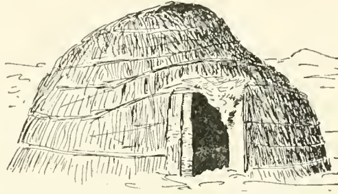
WICKYUP; PAI UTE FORM, OF TULE RUSHES; NEVADA. THERE IS GENERALLY AN OPENING AT TOP.
