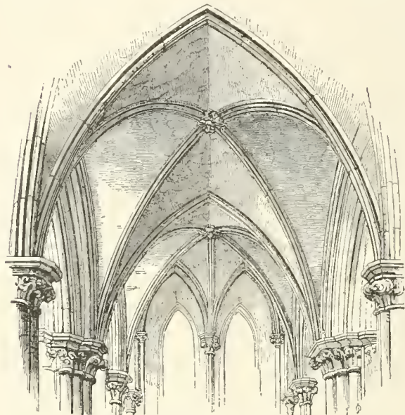
RIB, FIG. 1: EARLY RIBBED VAULTING WITH ONLY THE ESSENTIAL RIBS, VIZ., DIAGONAL RIBS (OGIVES) MEETING AT THE CENTRAL BOSS; TRANSVERSE RIBS SEPARATING THE VAULTING SQUARES; WALL RIBS (FORMERETS) ON RIGHT AND LEFT; THE COMPARTMENT IN THE DISTANCE IS, IN PART, IN SENPARTITE VAULTING; SALISBURY CATHEDRAL.
