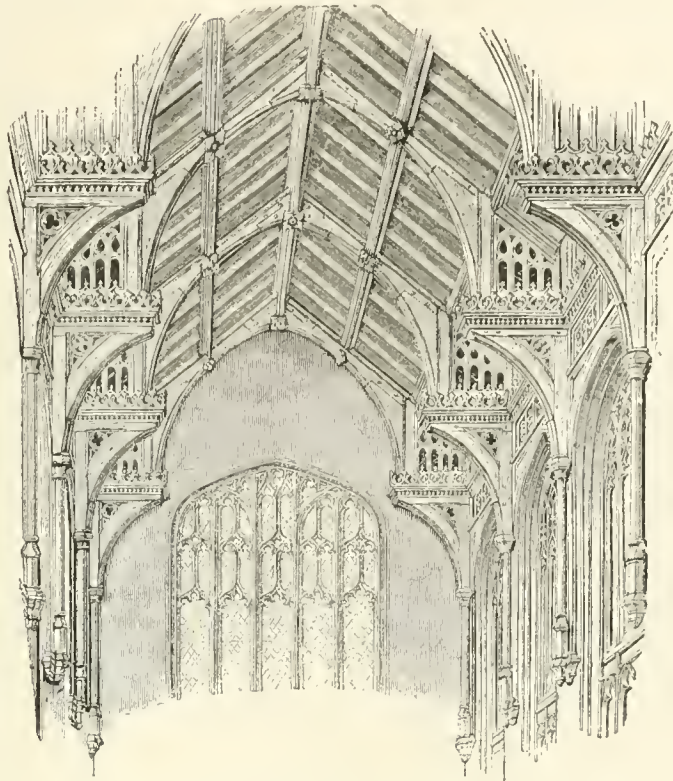
ROOF: ELABORATE HAMMER-BEAM CONSTRUCTION; S. STEPHEN'S CHURCH, NORWICH; c. 1480.
