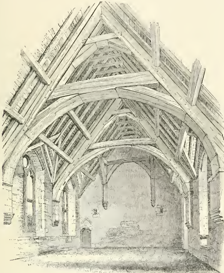
ROOF: WITH COLLAR BEAMS AND BRACES (KNEE RAFTERS), 13TH CENTURY; HALL OF STOKESAY CASTLE, SHROPSHIRE.
