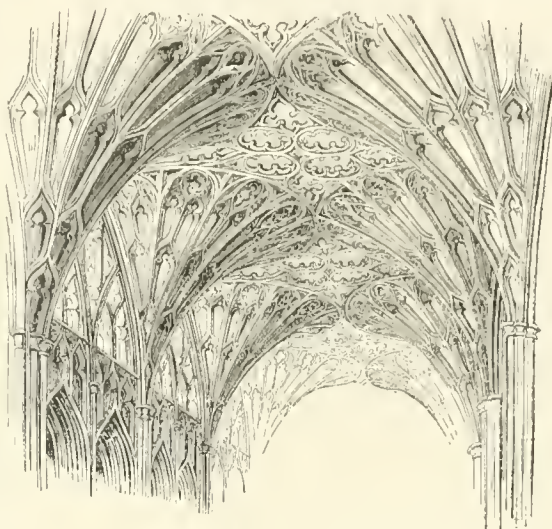
FAN VAULTING; CLOISTERS GLOUCESTER CATHEDRAL, c. 1450.
