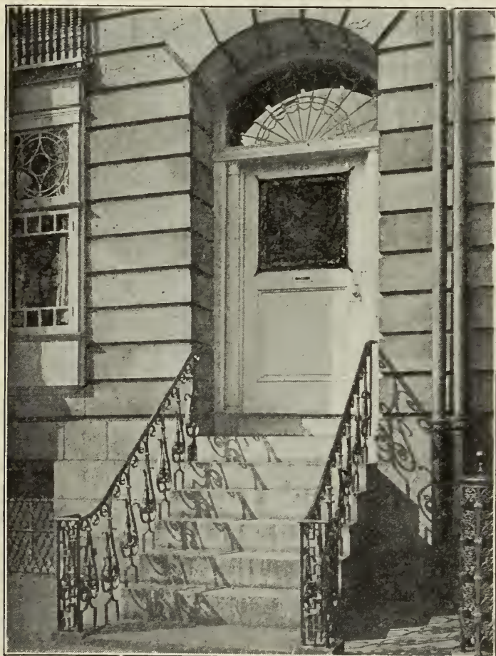
STEPS LEAD TO THIS DOORWAY
