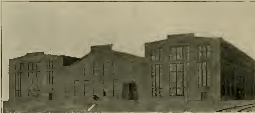
West End of Boiler, Machine and Erecting Shops.
