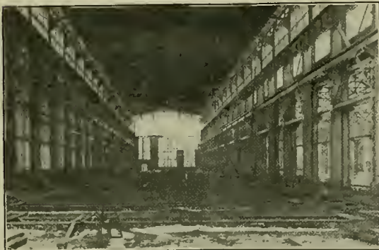
Construction View of Erecting Shop.
