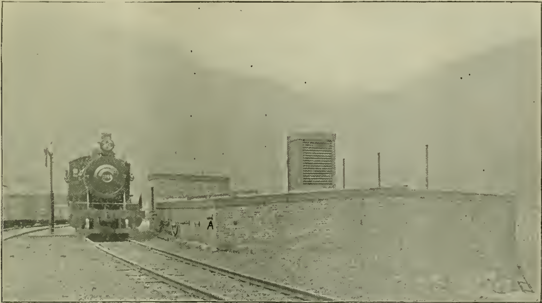
View of Station Showing Oil Burner Engine in Position Alongside Standpipe for Taking Oil. Oil Storage Station—Boston & Maine Railroad.
