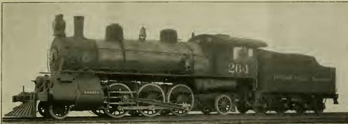
"Lake Shore" Type Tandem Compound Freight Locomotive—Chicago Great Western Railway.
