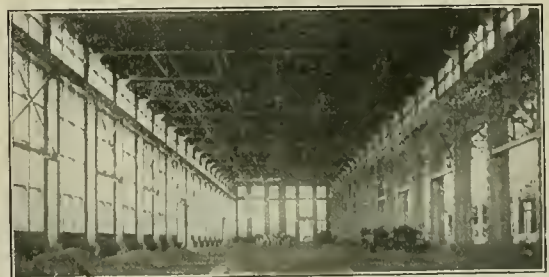
Interior View of Boiler Shop.
