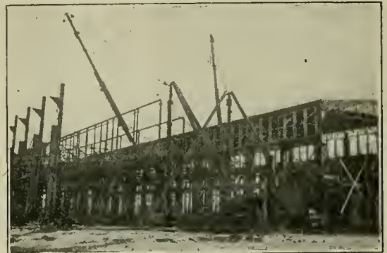
Exterior Construction View of Machine Shop.
