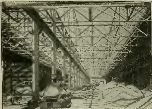
Interior Construction View of Machine Shop.
