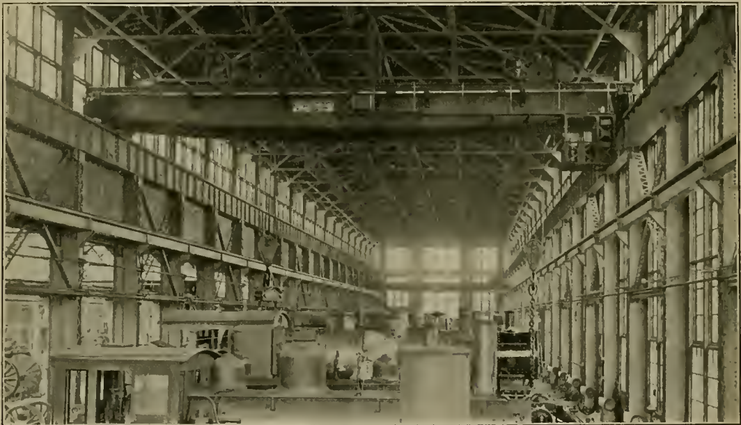
General View of Erecting Shop, Showing 10-Ton and 100-Ton Cranes. (Air Delivery Outlets Appearing on Floor at Right.)
