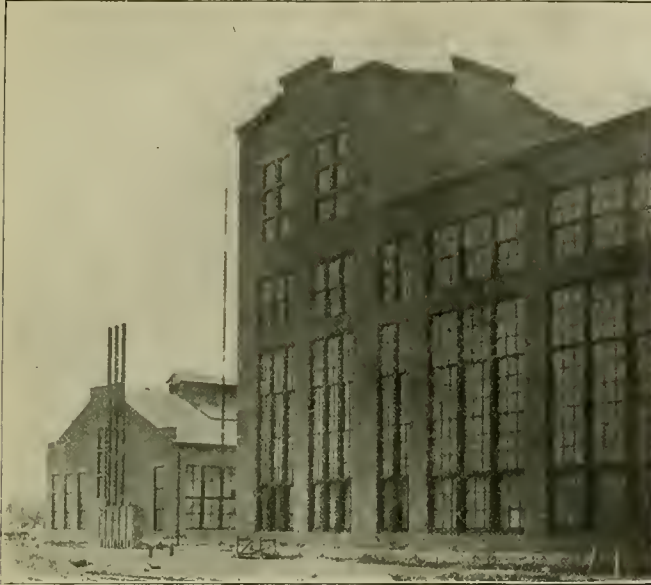
Northeast Corner of Boiler Shop, Showing Riveting Tower.
