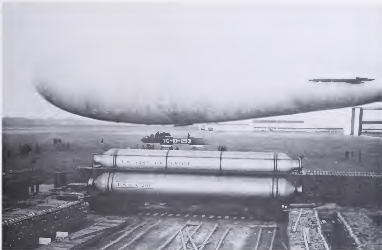
Prior to the introduction of this tank car, the transportation of helium in canisters by truck and rail was cumbersome and costly, November 1926. In the background the TC-10-253, still carrying its TC-8 marking, is landing.
