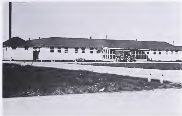
Post hospital. According to the field's first physician, Dr. Ernst C. Asbury, the hospital offered little privacy. Patients watched as others received treatment. Insufficient beds, medicines, operating room equipment, and personnel were major problems until the spring of 1918.
