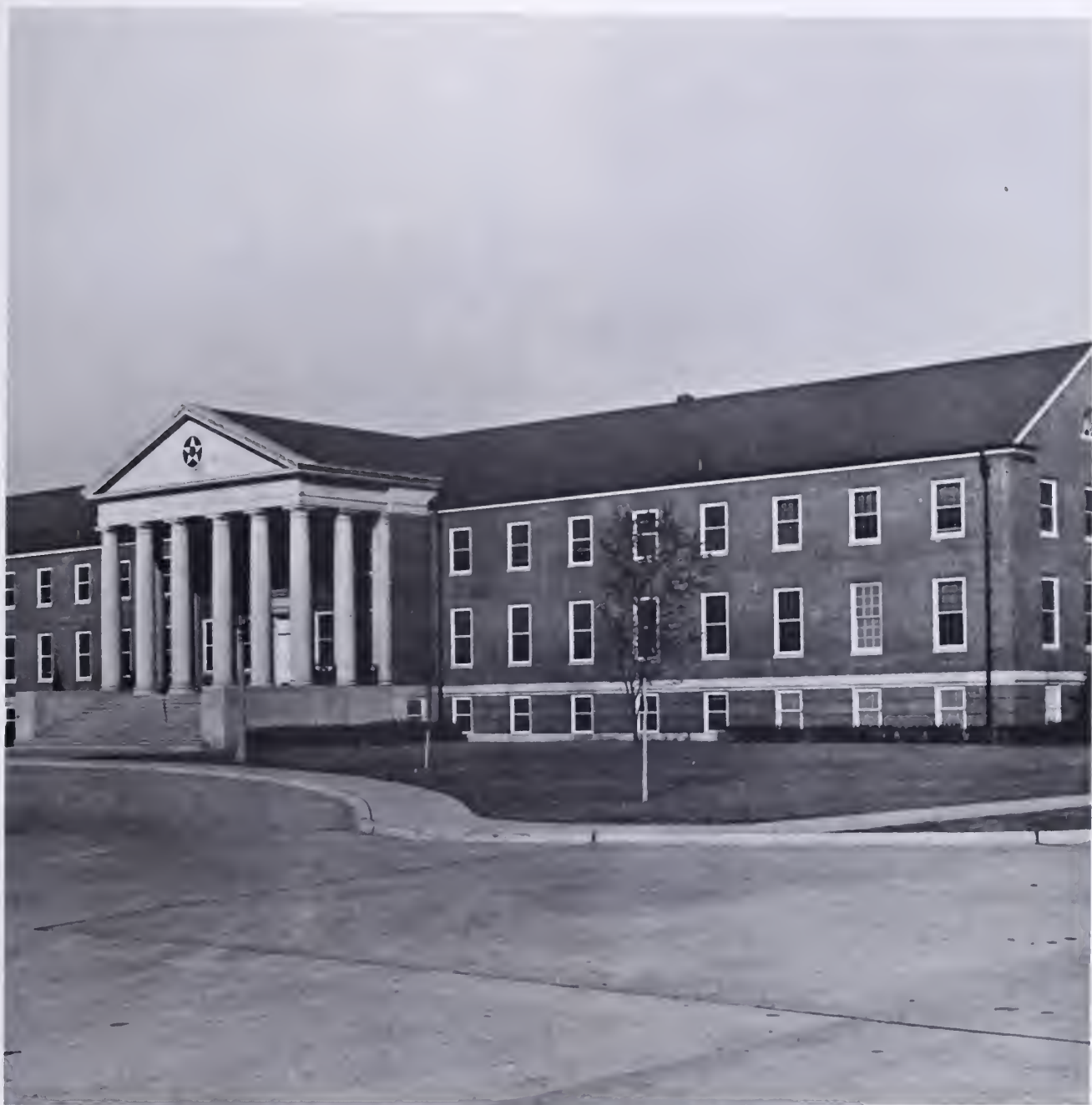
Titled General Headquarters Air Force, the elaborate P-3 never served as the headquarters for the Air Corps' air combat arm, November 1940. During the war the $183,300 building contained the post headquarters.
