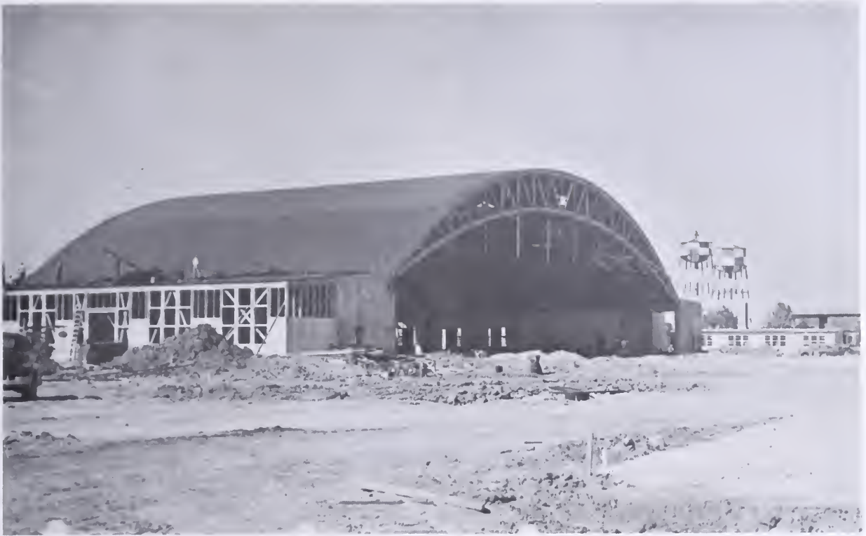
The readiness hangar (presently Hangar No. 3) under construction, October 1952.
