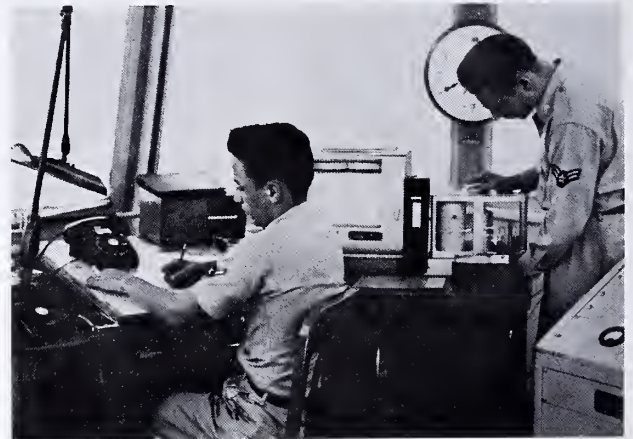
Representative observation site (ROS) on top of Hangar No. 1, September 1961. Two weather observers prepare a “special” observation. The observer on the left is encoding the elements of the observation on the WBAN Form 10 while the observer on the right checks the barograph for the current pressure trend and reads the altimeter setting from the aneroid barometer (small box).
