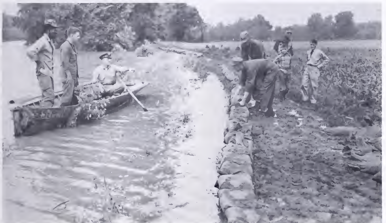
Reinforcing weak spots along the levee, July 1951. The Mississippi crested at 40.28 feet at St. Louis. So great was the need for volunteers that over 900 airmen assisted with flood control operations. On 17 July, three C-124 Globemasters each loaded with 50,000 sandbags landed for the first time at Scott. Other major floods in this period occurred in 1943, 1946, and 1947. Over the years, the base has lent a helping hand during many natural disasters.
