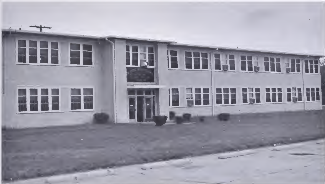
Headquarters 932nd Troop Carrier Group in Building 3650, September 1963.
