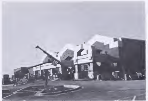
Scott's new commissary under construction, 1987.
