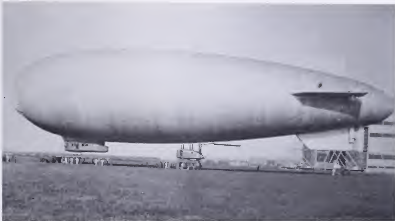
Beginning its second flight on 15 January 1926. The RS-1 had a maximum speed of 50 mph and a range of 2,588 miles.
