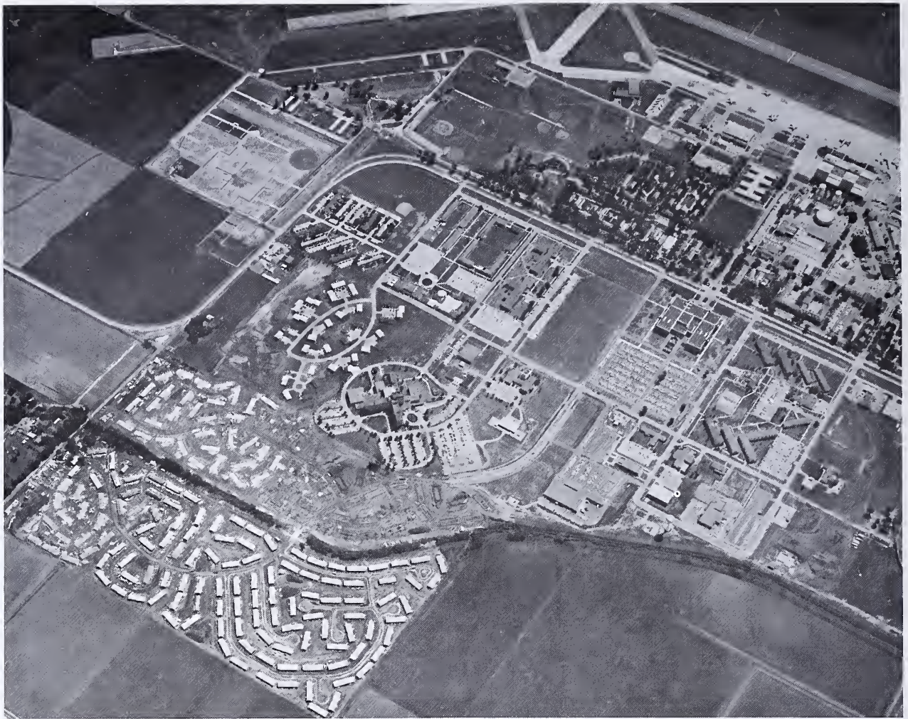
This aerial photograph shows most of the new construction, circa 1973.
