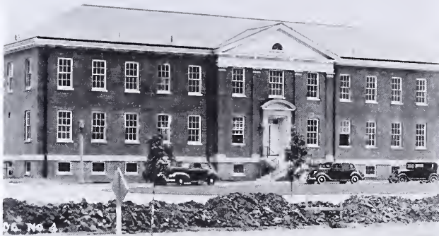
The field's hospital remained the World War I structure for twenty-three years until the completion of this brick building (Bldg. P-4). The new hospital cost $219,500. It was soon inadequate for World War II requirements.
