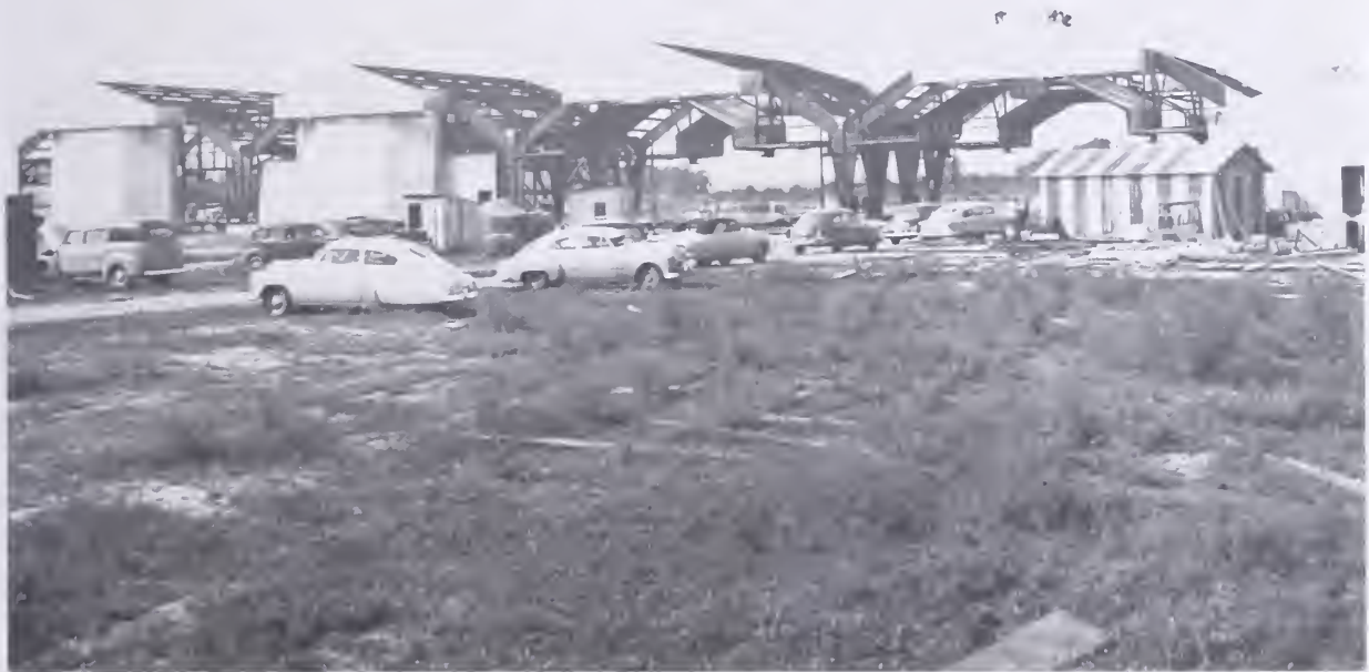
Framework of the new alert hangars, August 1952.
