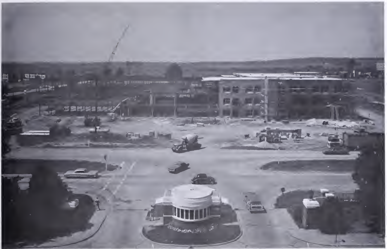
Headquarters MAC under construction, 36 percent complete by August 1970.
