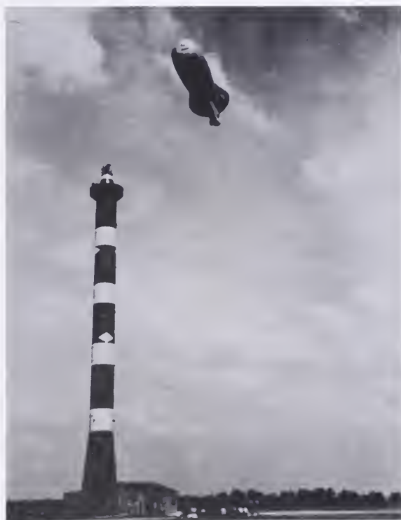
An observation balloon being moored to Scott's $85,000 mast, September 1928. Docking a LTA craft was not a complicated maneuver but did require precision and good judgment. Regardless of wind velocity, Scott's mast was designed to moor all types of airships. While moored, a ship could be serviced with water, fuel or helium, which was piped to the top of the tower.
