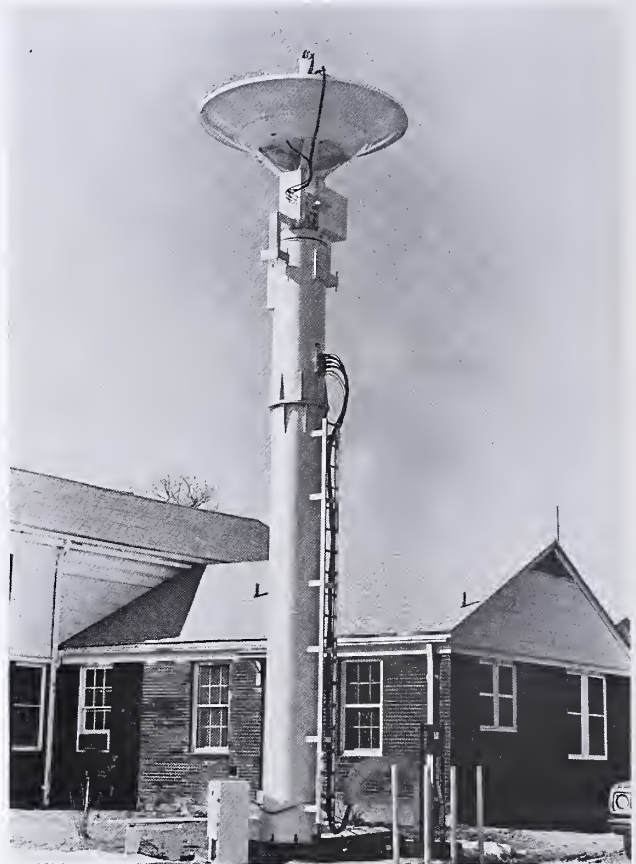
The SARSAT (Search and Rescue Satellite-Aided Tracking) satellite receiving antenna at Scott, 1982.
