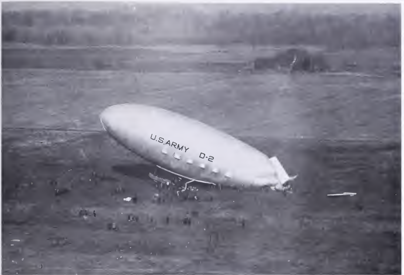
Partial collapse of the D-2 airship, circa 1922. Although a leak in a gas cell or a loss in pressurization could result in an accident, the airship was as good as new with a little patching. Airship mechanics were quick to make this point with their heavier-than-air counterparts.
