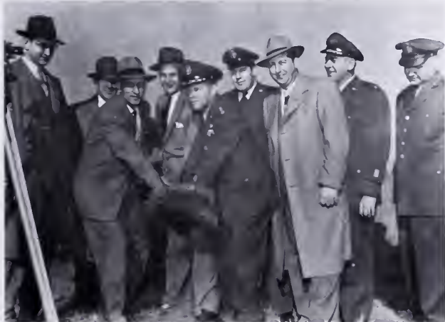
Breaking ground for the $8.5 million Wherry Housing project, 5 January 1951. Major General Robert W. Harper, right, and Wesley Bloomer, president of the Belleville Chamber of Commerce, turned the first spade of earth.
