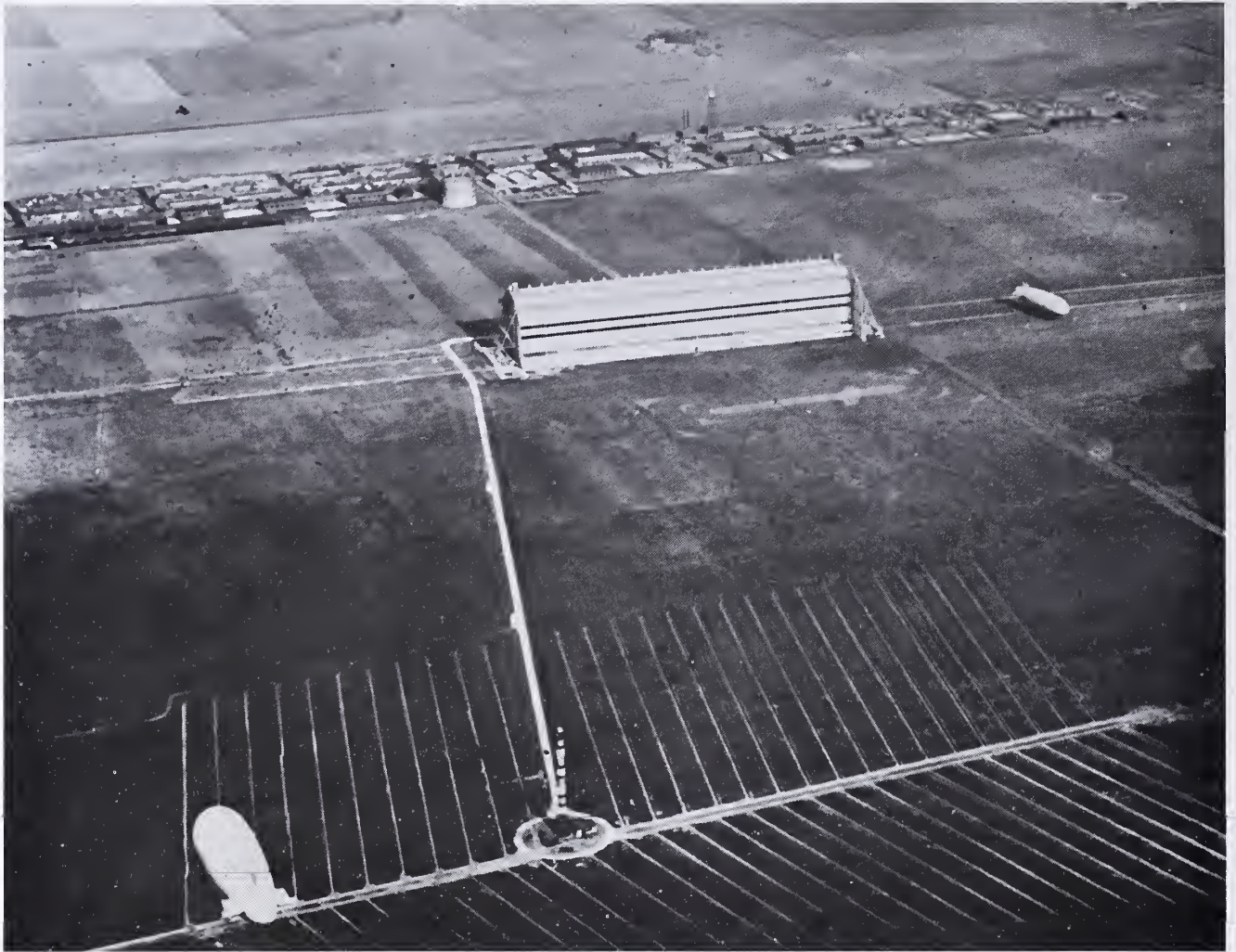
Looking west, full view of Scott's LTA facilities, circa 1927. The parallel lines by the mast were drainage tiles. Two docking rails extended 1,000 feet from each end of the airship hangar.
