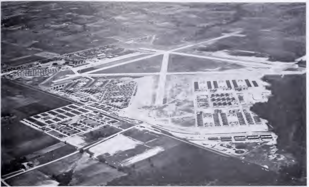
Full view of Scott Field with its four runways, 1943. The runway work cost $1 million.
