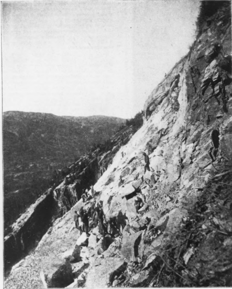
FIG. 3.—BEGINNING WORK ON FISK'S CUT, TUNNEL MOUNTAIN; WHITE PASS & YUKON RY.
