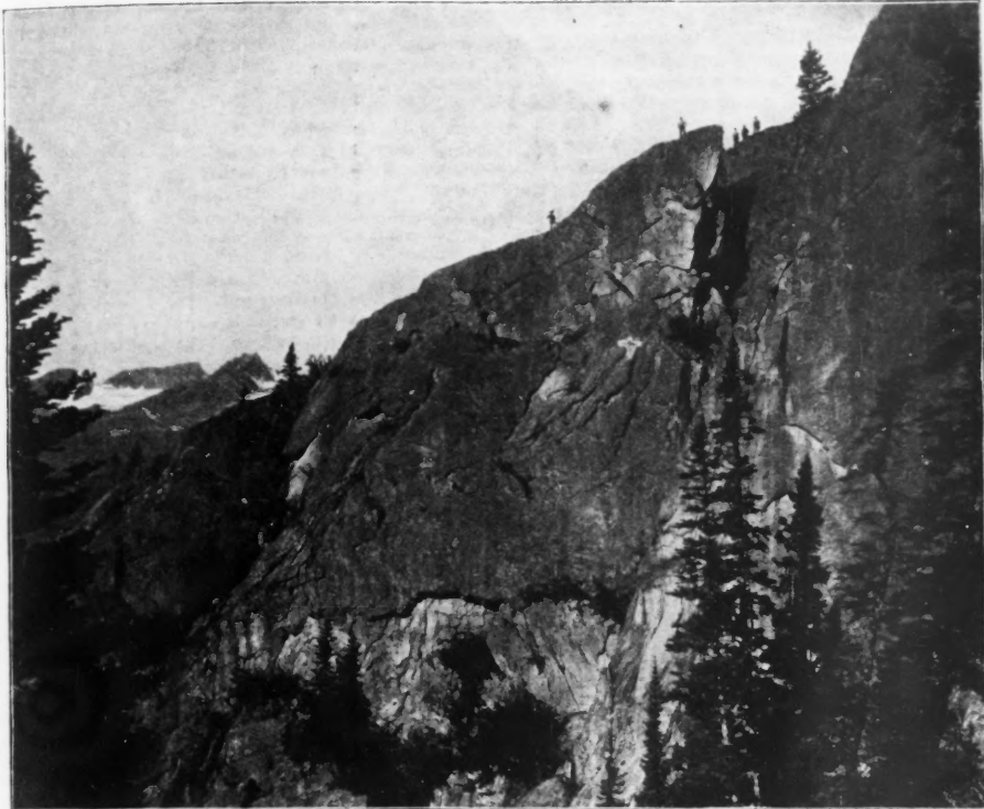
FIG. 4.—SITE OF TUNNEL.
