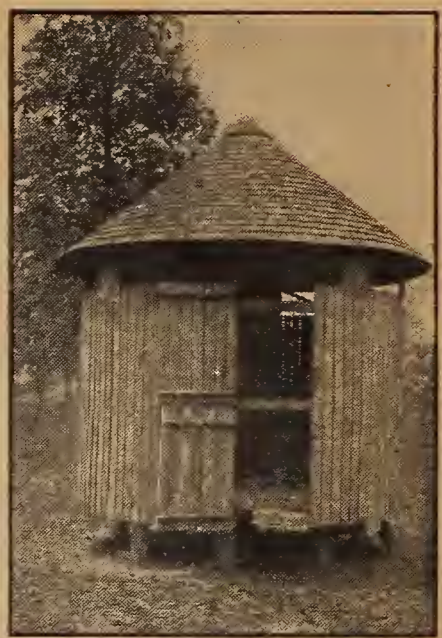
Fig. 2—Showing the doorway and ventilator of the barrel crib
