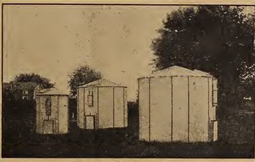
Fig. 3—Steel bins for small grains
