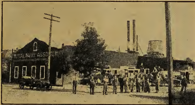
The milk plant, wagons, and employees
