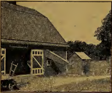
The fireproof gasoline engine house is outside of the barn
