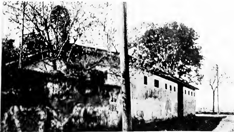
KITCHEN AND WALL MADE OF "TABBY" The Sams' Home, Beaufort, now the Crofut House
