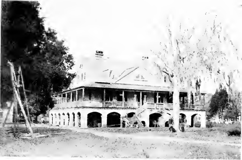
"DEAN HALL," COOPER RIVER, BELOW THE TEE
