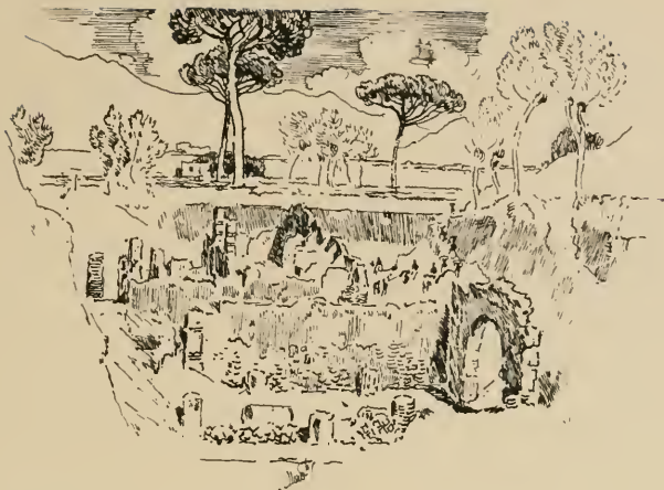
New Excavations, Pompeii
