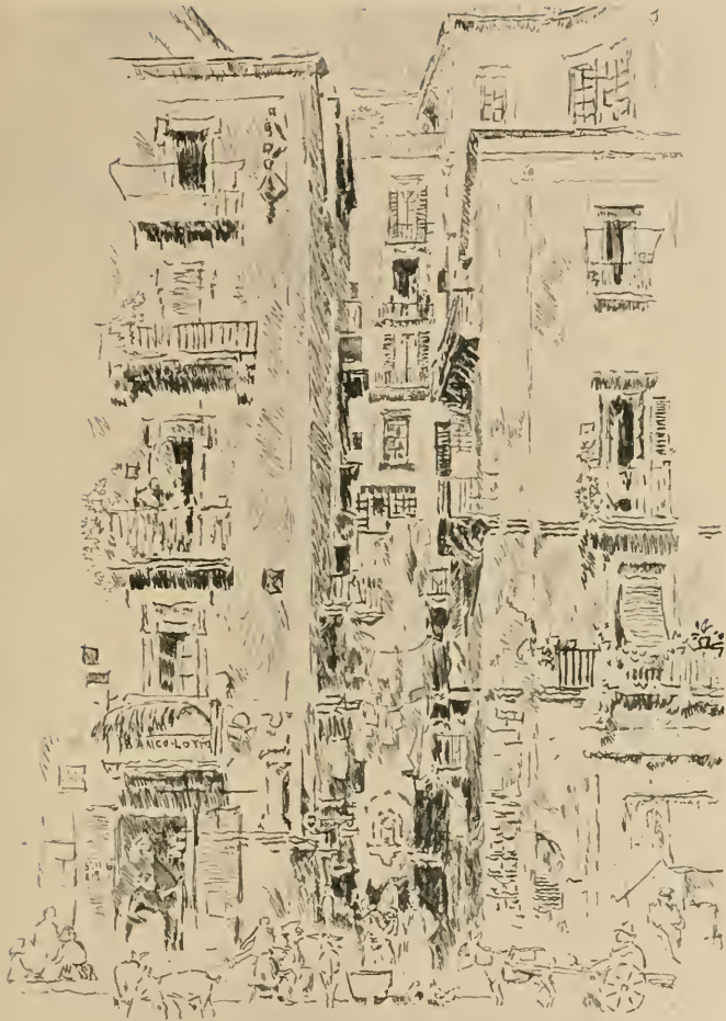
Santa Lucia (now being demolished), Naples
