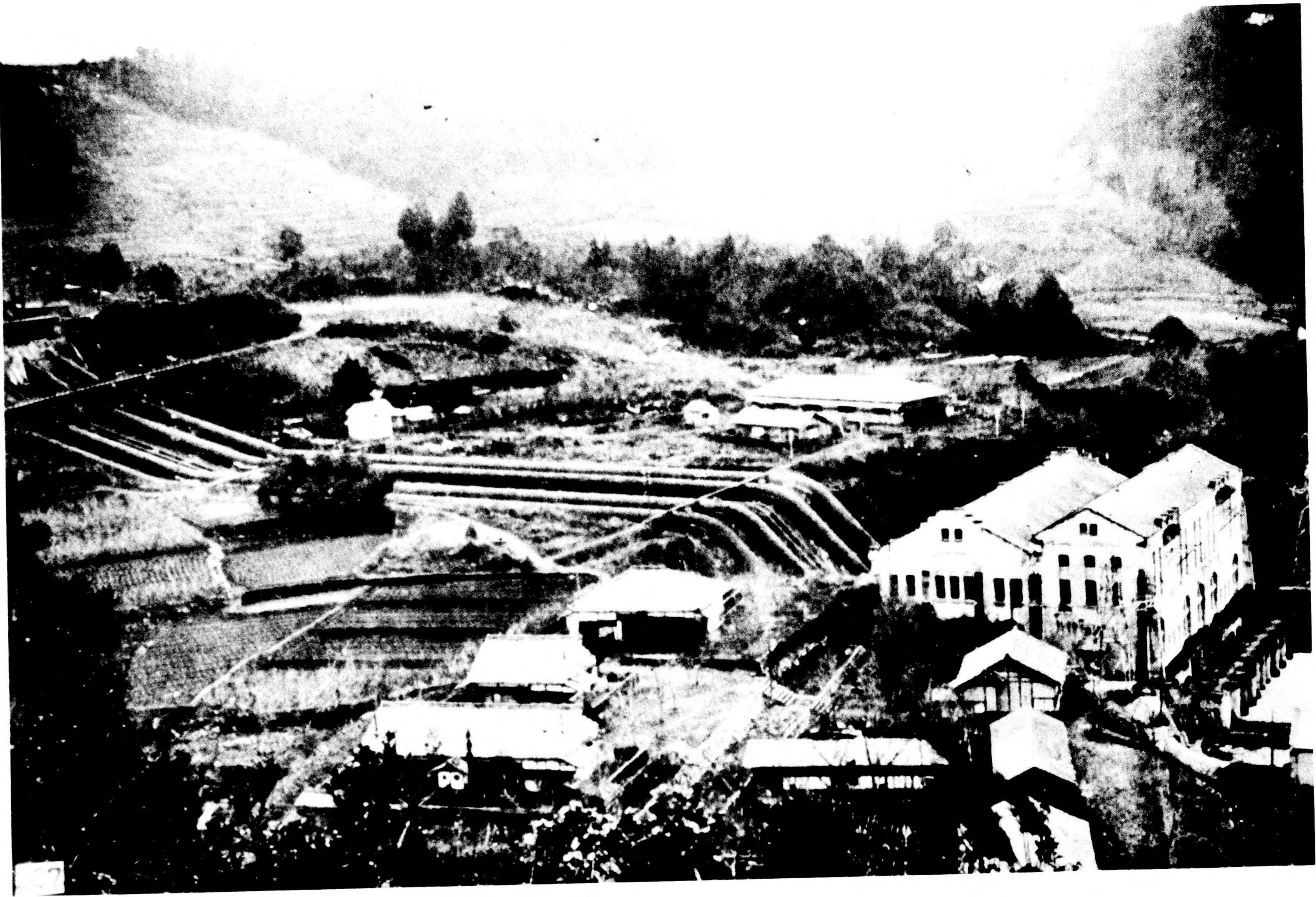
Photograph No. V-95 Yaotsu Hydro Plant
