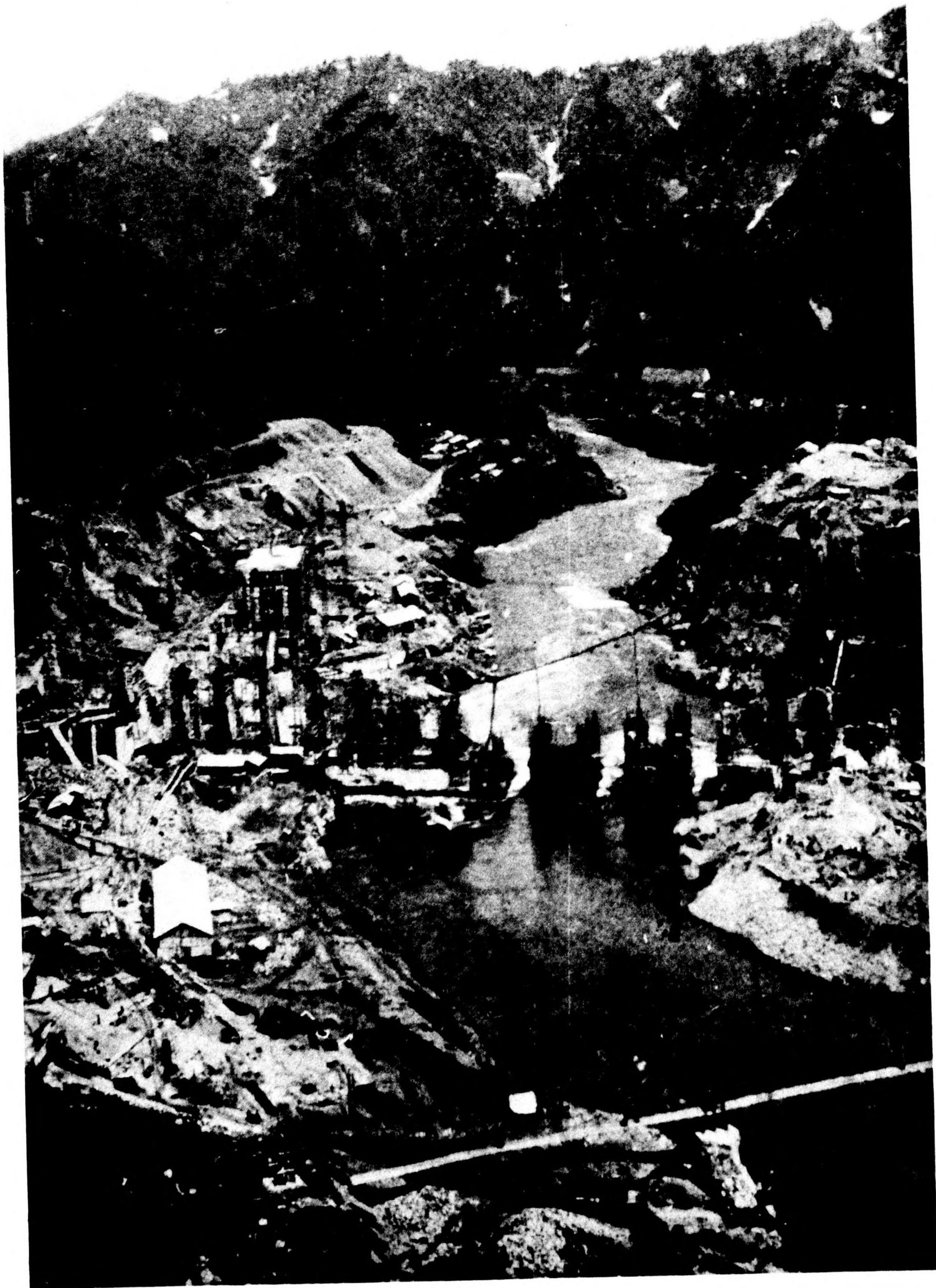
Photograph No. V-66 Toyomi Hydro Plant and dam under construction
