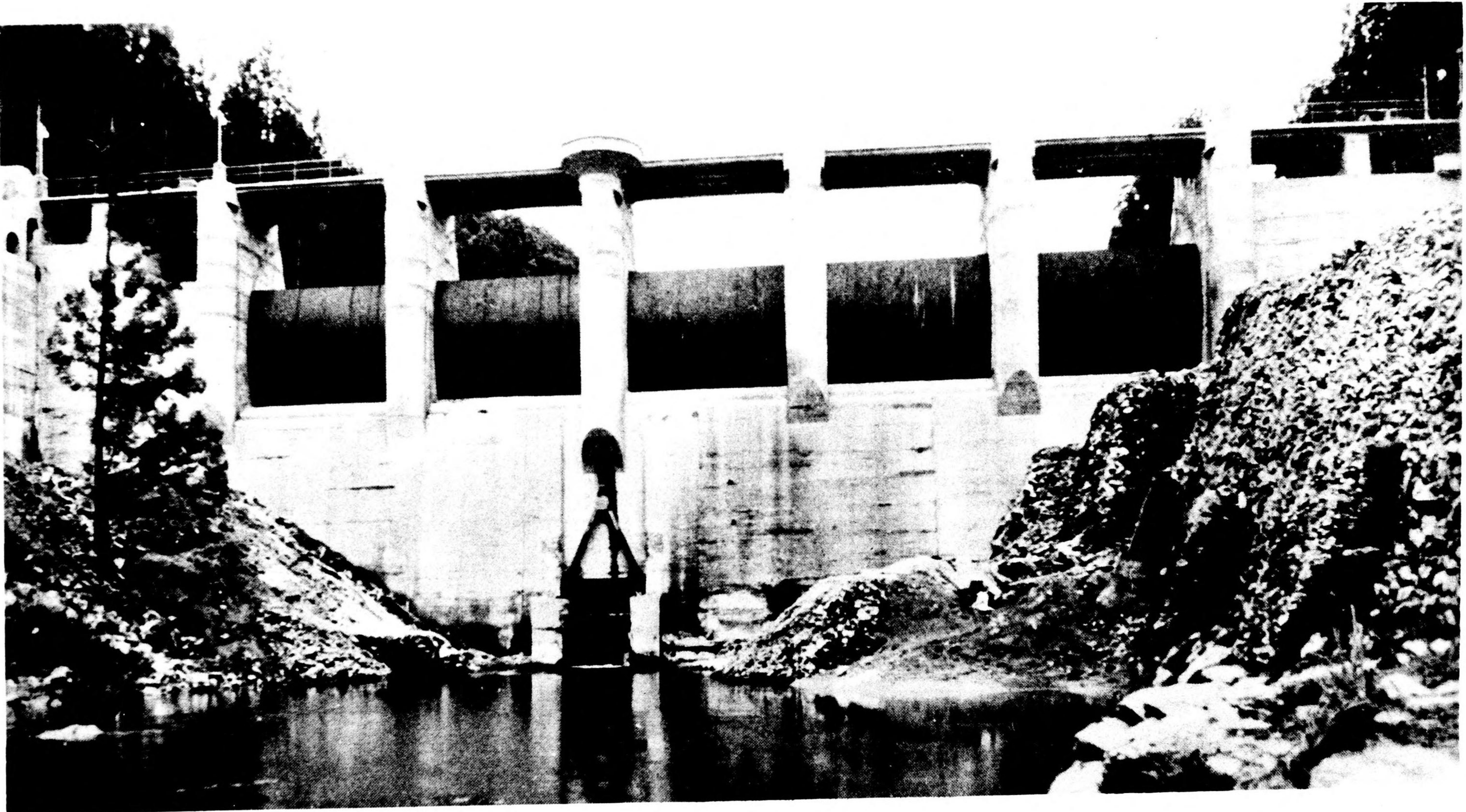
Photograph No. V-88 Tsuzurao Dam of the Ujigawa Denki KK Wada Hydro Plant in 1937
