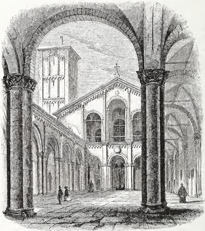
CHURCH OF S. AMBROGIO, MILAN, A.D. 835, (SHEWING THE ATRIUM AND WEST FRONT).
