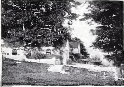
Maxfield Parrish's Residence, Cornish, N. H. Stained with Cabot's Shingle Stains
