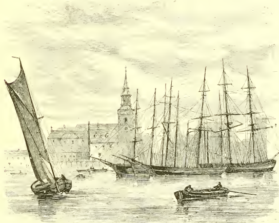
ROTHERHITHE CHURCH: TUNNEL FIER.
