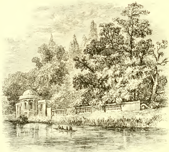
WATER PAVILION AT SION HOUSE.
