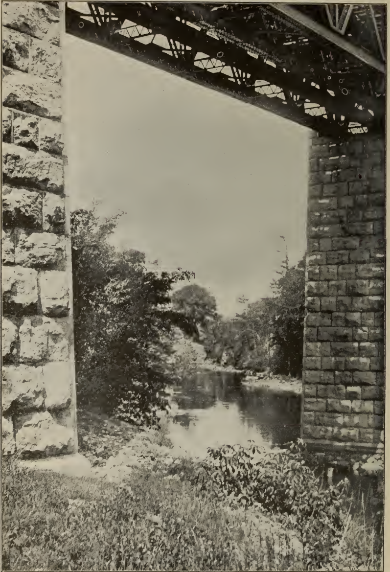
View through Arch of Railway Bridge, Kingston Mills
