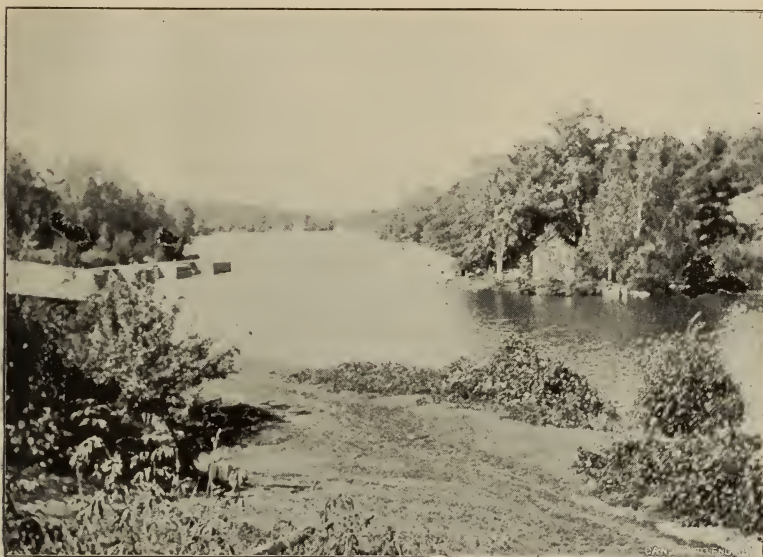
LOOKING NORTH FROM FOSTER'S LOCK
