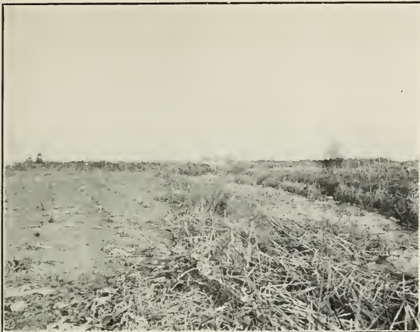
FIG. 1.—MAIN DITCH LEADING TO SLUICE 4. [Example of a choked ditch.]
