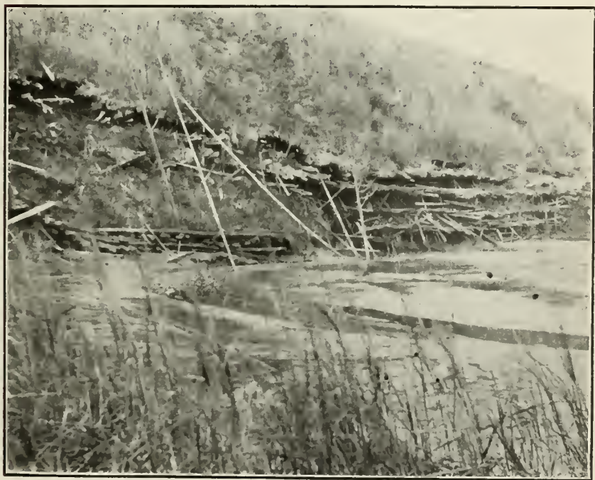
FIG. 2.—LAND SIDE, SHOWING LAYERS OF BRUSH AND ORDINARY HEIGHT OF INTERIOR WATER.
