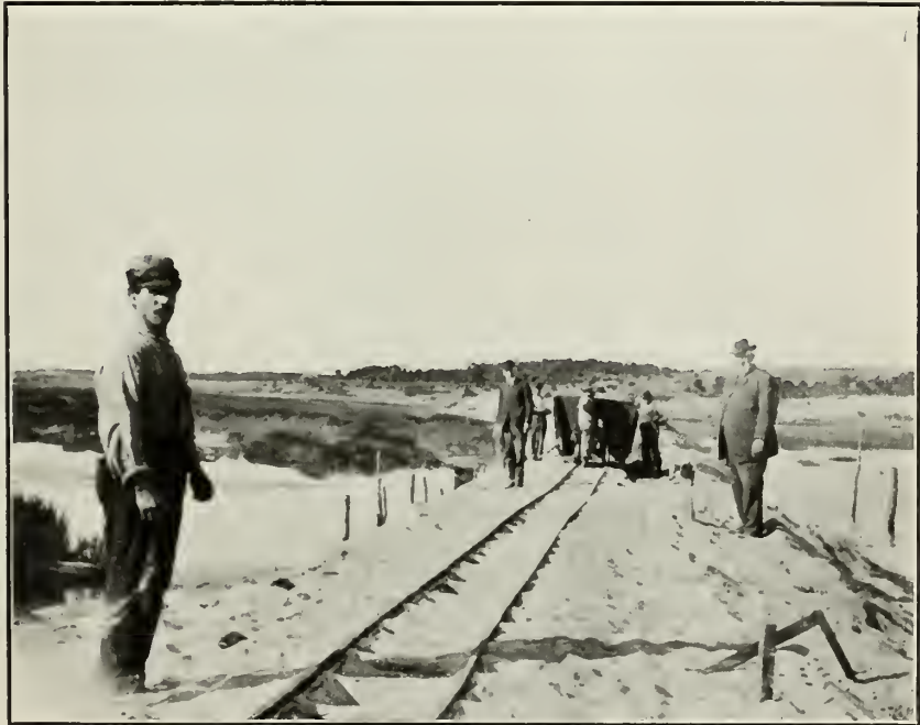
FIG. 2.—DIKING OPERATIONS, SHOWING METHOD OF PLACING MATERIAL. DIKED LANDS AT WELLFLEET, MASS., SEPTEMBER 22, 1910.
