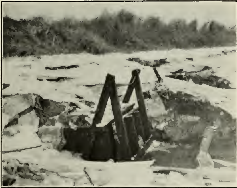
FIG. 2.—SLUICE 8, SHOWING GATE SLIGHTLY OPEN, HOW THE WEIGHT OF THE GATE RETARDS THE DISCHARGE AND THE LIABILITY TO INTERFERENCE FROM ICE.
