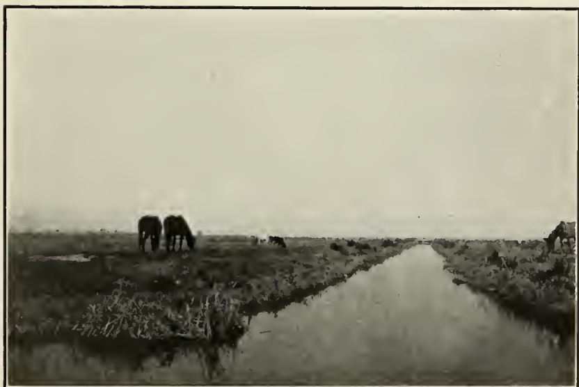
FIG. 2.—EXAMPLE OF A LATERAL DRAINAGE DITCH.
