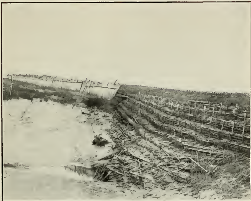
FIG. 1.—WATER SIDE, SHOWING METHOD OF PICKET AND HEADING BRUSH PROTECTION, AND ON THE LEFT, PLANK PROTECTION FOR "RUNNING DIKE."
