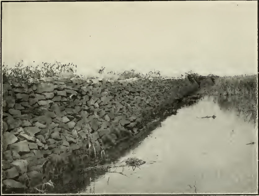
FIG. 1.—ROCK-FACING FOR PROTECTION OF LEVEE AND FORESHORE AT HALF-TIDE LEVEL, ST. GEORGES MARSH CO., NEW CASTLE COUNTY, DEL., NOVEMBER 1, 1909.
