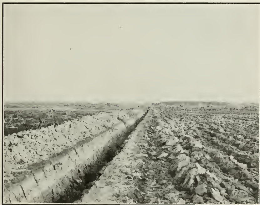
FIG. 2.—LATERAL DITCH NEAR SLUICE 3. [Example of a clear ditch.]
