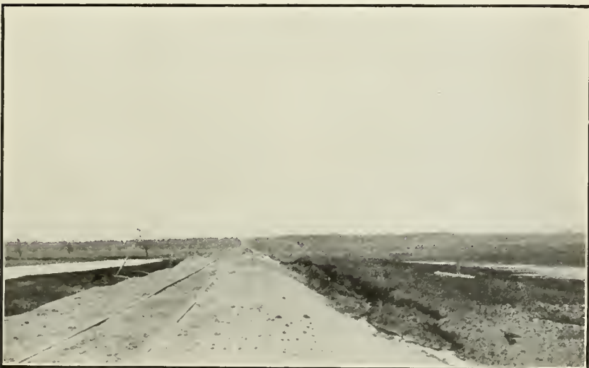
FIG. 2.—DURING NEW CONSTRUCTION WORK, DECEMBER, 1903.
