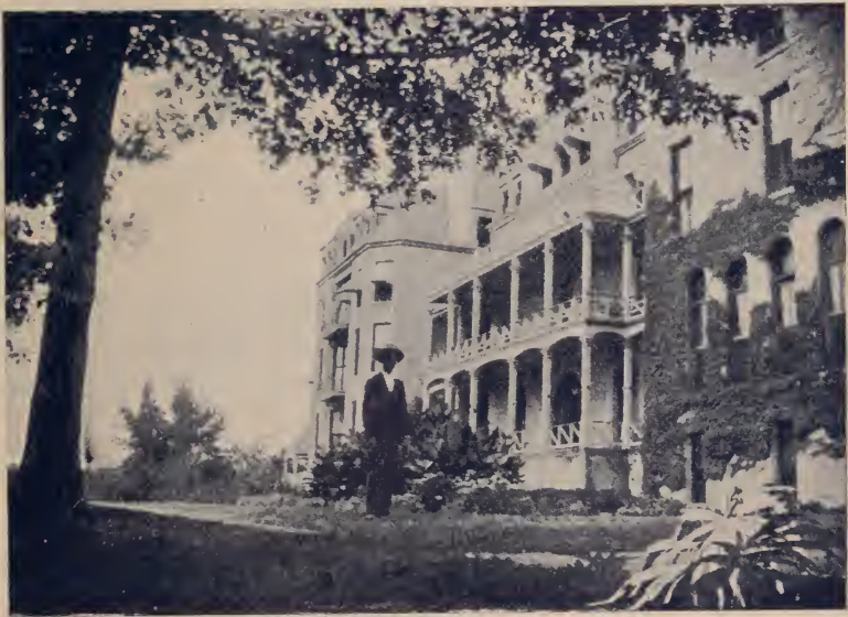
A CORNER OF THE GROUNDS. CRESCENT HOTEL.
