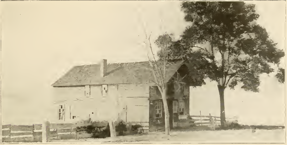
Peter Runquists' old blacksmith shop
