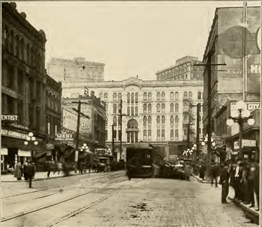
THIRTY YEARS OF PROGRESS OCCIDENTAL AVENUE LOOKING NORTH TO YESLER WAY
