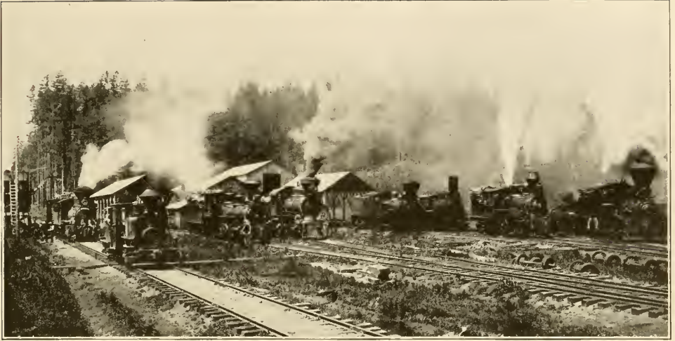
THE RAILROAD YARD OF A LUMBER CAMP
