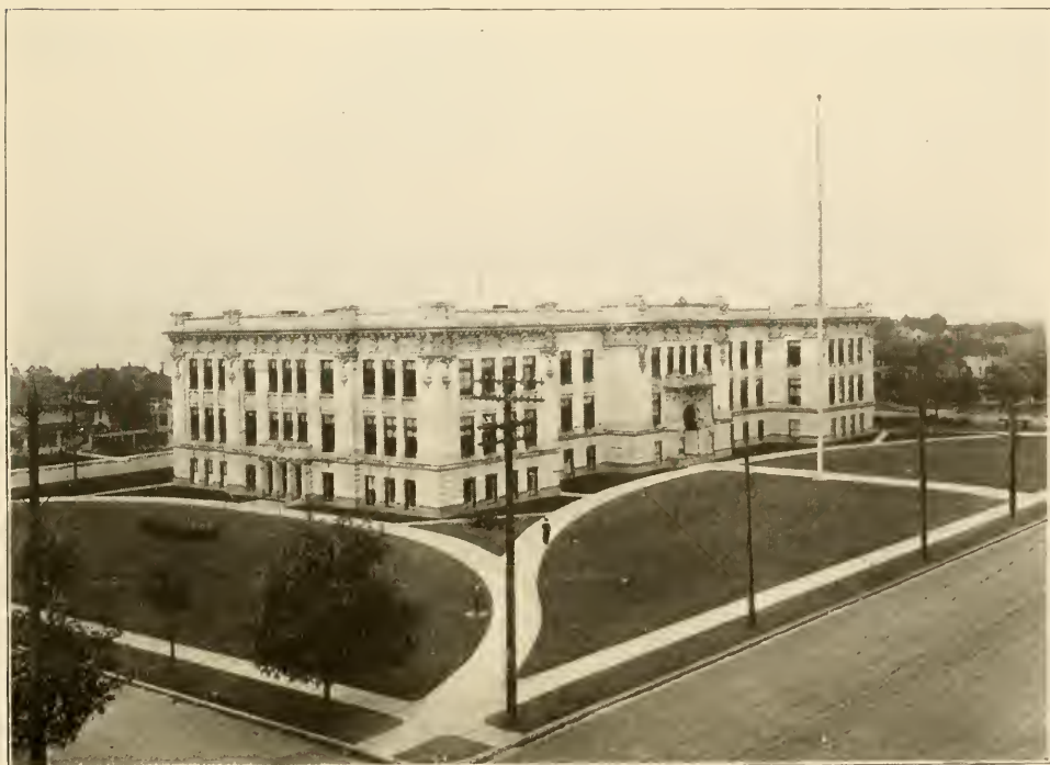
EVERETT HIGH SCHOOL BUILDING
