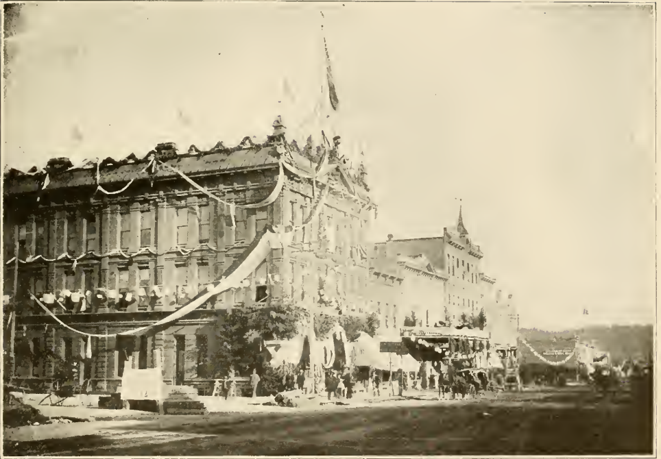
TACOMA CELEBRATING THE COMPLETION OF THE CASCADE DIVISION OF THE NORTHERN PACIFIC RAILWAY, JULY 6, 1887
