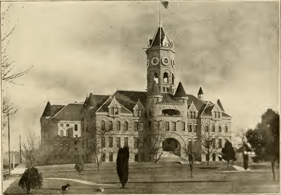
STATE CAPITOL BUILDING, OLYMPIA
