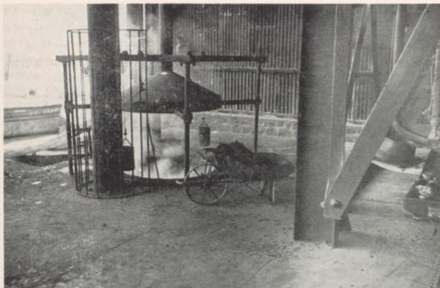
*Lead furnace in insoluble anode plant of copper smelter*
