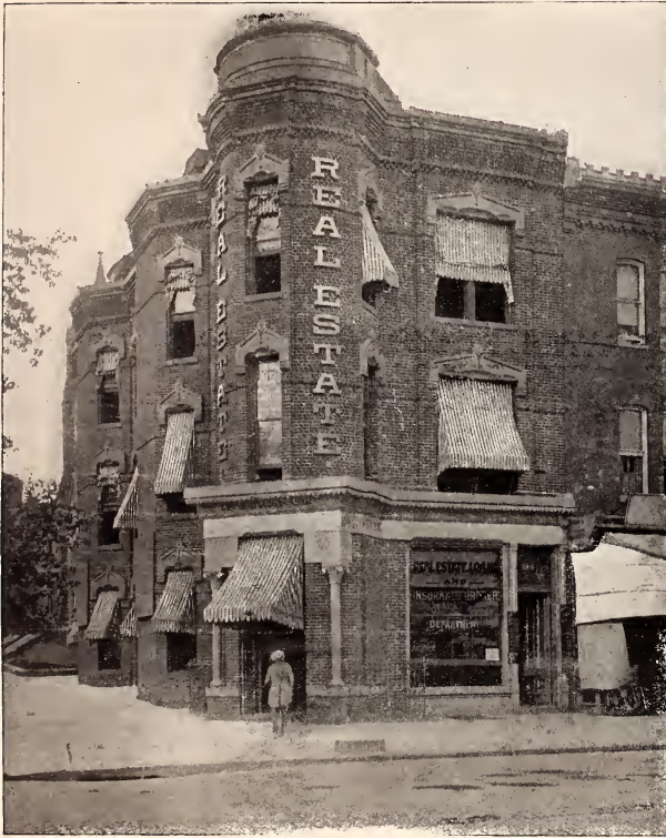
OFFICE OF D. I. MURPHY, HOLTZMAN BUILDING, WASHINGTON, D. C.
