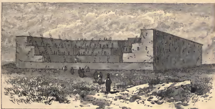
RESTORATION OF THE PUEBLO HUNGO PAVIE.
