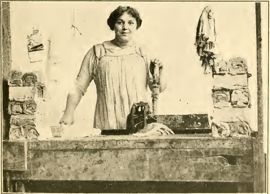
FIG. 2.—MAKING COD BRICKS.
