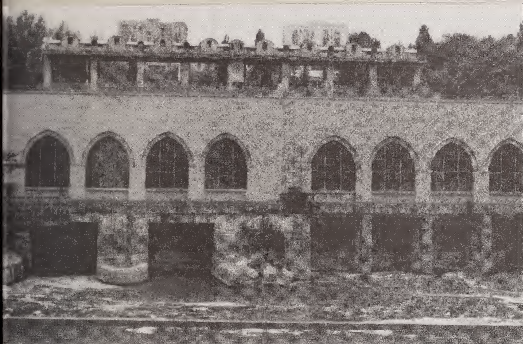
Hydroelectric station on Georgian Military Highway between Tbilisi and Mtskheta
