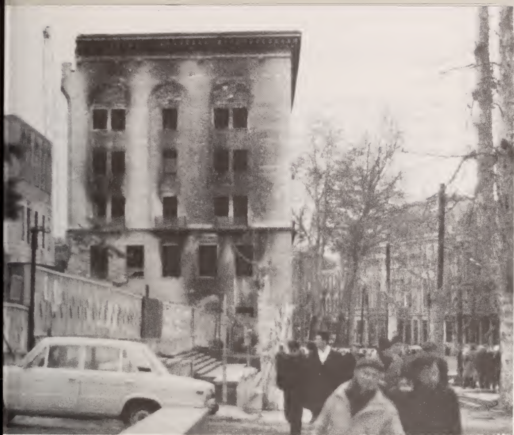
Burned-out headquarters building of Georgian Communist Party, Tbilisi, 1992
