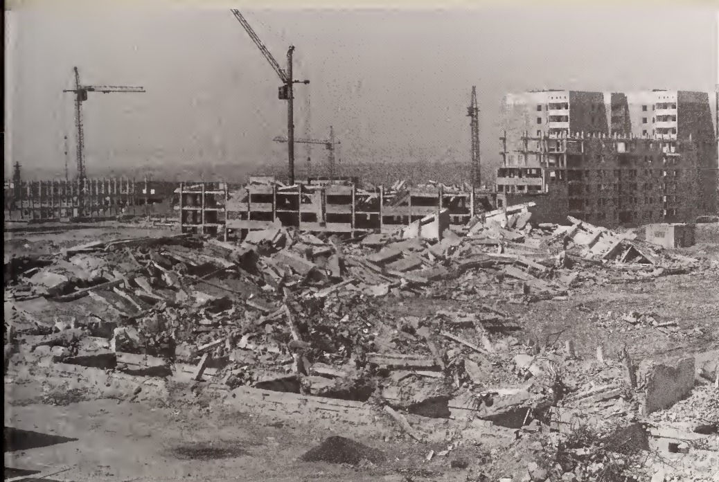
Damage to apartment buildings in Leninakan (present-day Gyumri) caused by 1988 earthquake Courtesy John Filson
