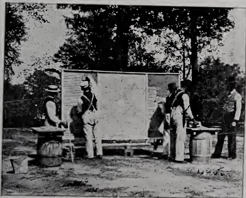
LESSON IN PLASTERING.
