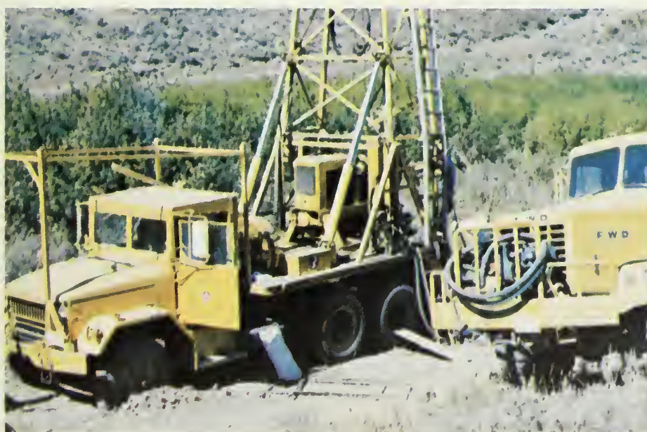
View of drill rig on drill hole, DH-3. This hole sets in the bottom of a canyon and encountered artesian water.
