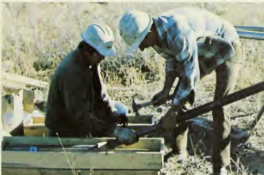
Drillers removing core from core barrel on drill hole, DH-3.
