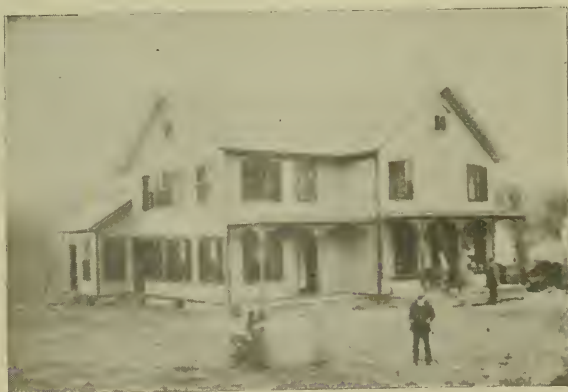
RESIDENCE AND STORE OF FRED H. CHASE, SOUTH KENT.
