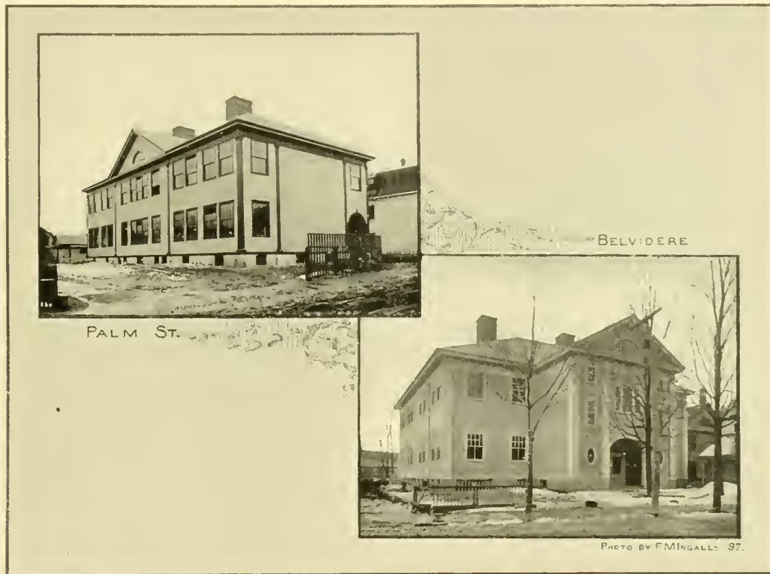
SCHOOL HOUSES, ERECTED IN 1860-67.
