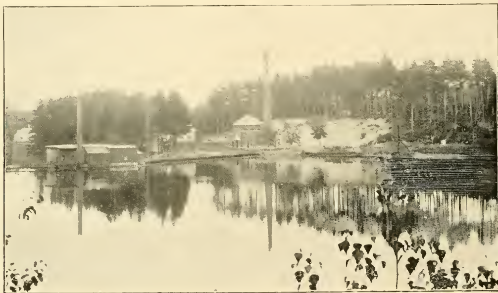
PENNICHUCK WATER WORKS' PUMPING STATION.
