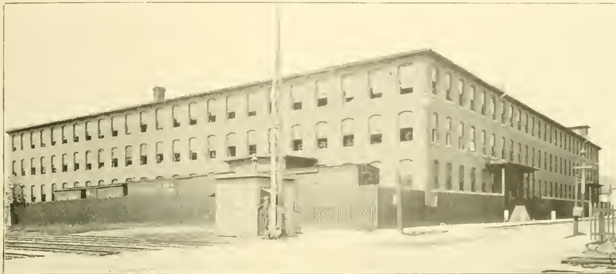
ESTABROOK-ANDERSON SHOE FACTORY. (PALM STREET VIEW)
