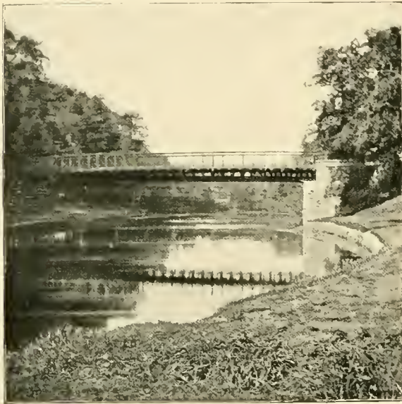
THE OLD IRON BRIDGE OVER THE NASHUA AT CANAL AND BRIDGE STREETS.
