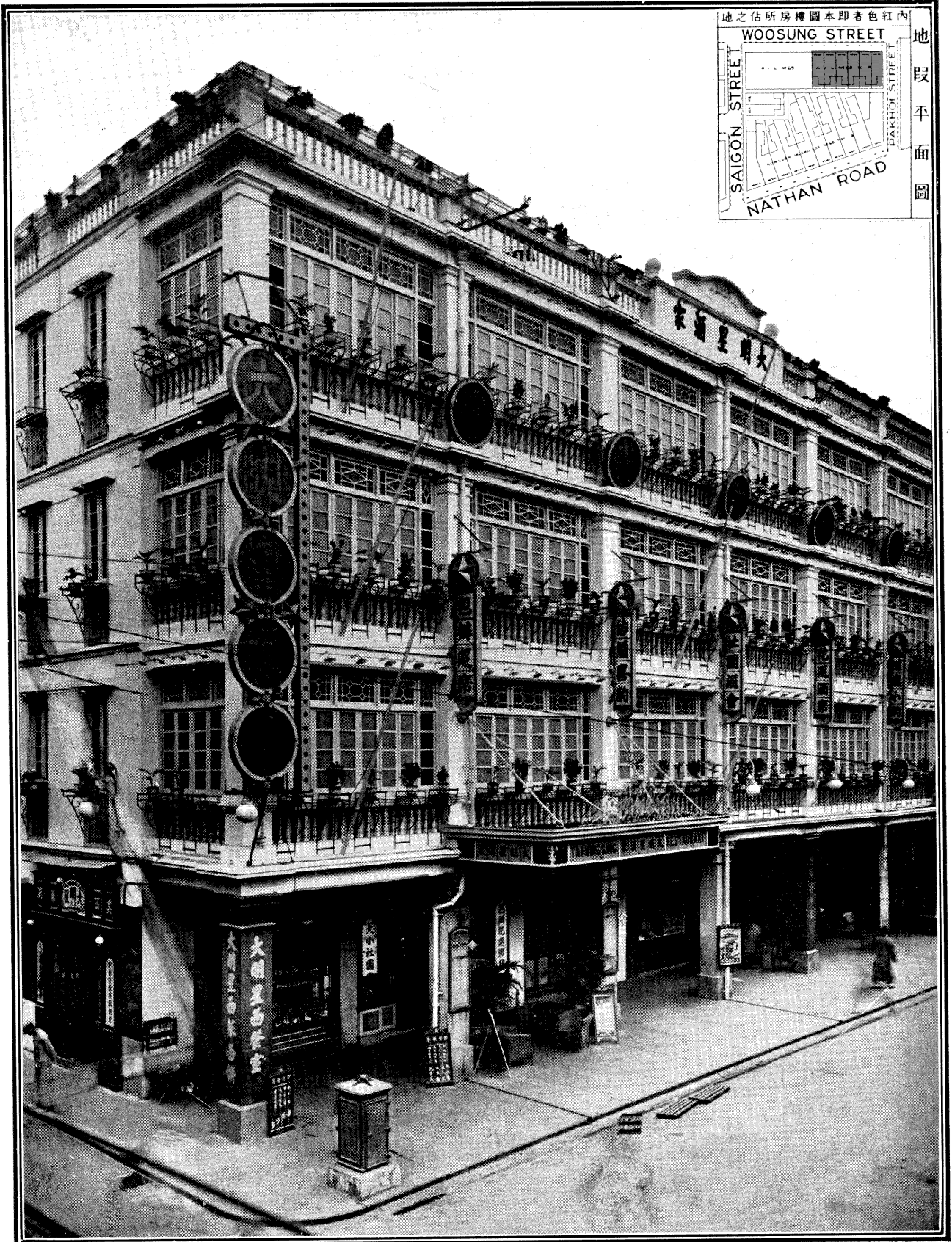
THE COMPANY'S PROPERTY (30-40 WOOSUNG STREET, YAUMATI)
