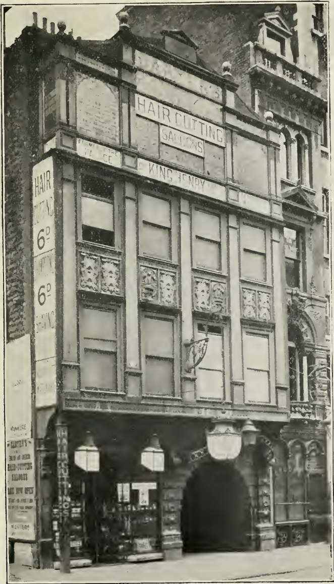
No 17 Fleet Street before Restoration.
