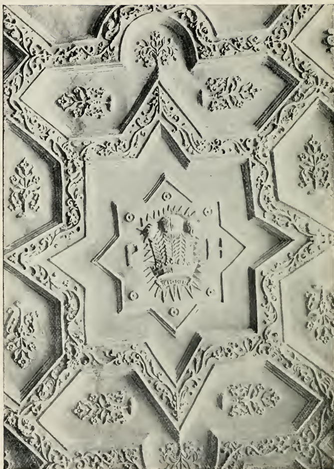
Plaster ceiling, No. 17, Fleet Street.
