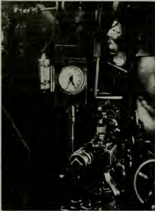
FIG. 5.—The Loco Valve Pilot in the Locomotive Cab.
