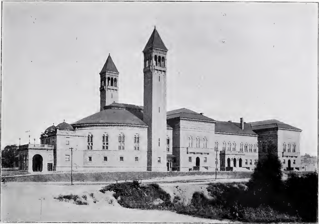
The Carnegie Art Gallery, Pittsburgh, Pennsylvania. Messrs. Longfellow, Alden and Harlow, Architects.
