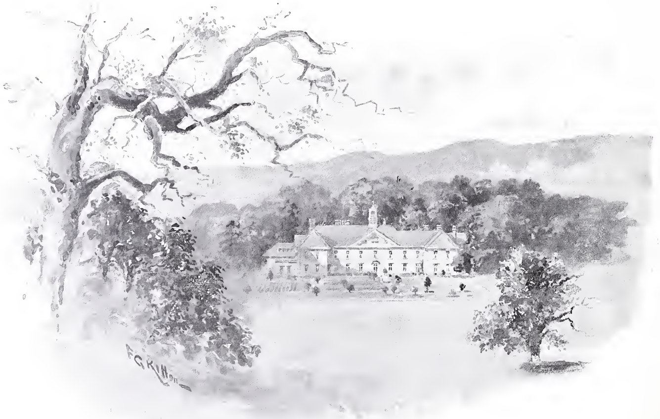
The Priory, Reigate.
