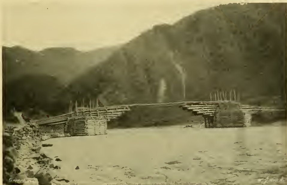
FIG. 82.—BRIDGE OVER TOW RIVER.
