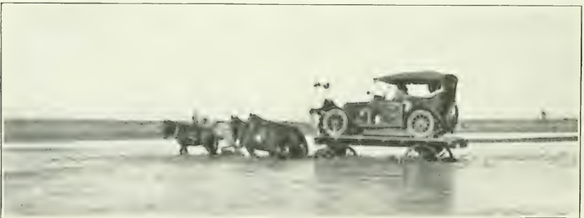
CROSSING THE GILA RIVER AT FLORENCE, ARIZONA.
