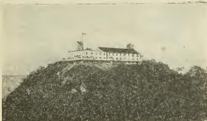
The Prospect House Looks Down from Mt. Holyoke
