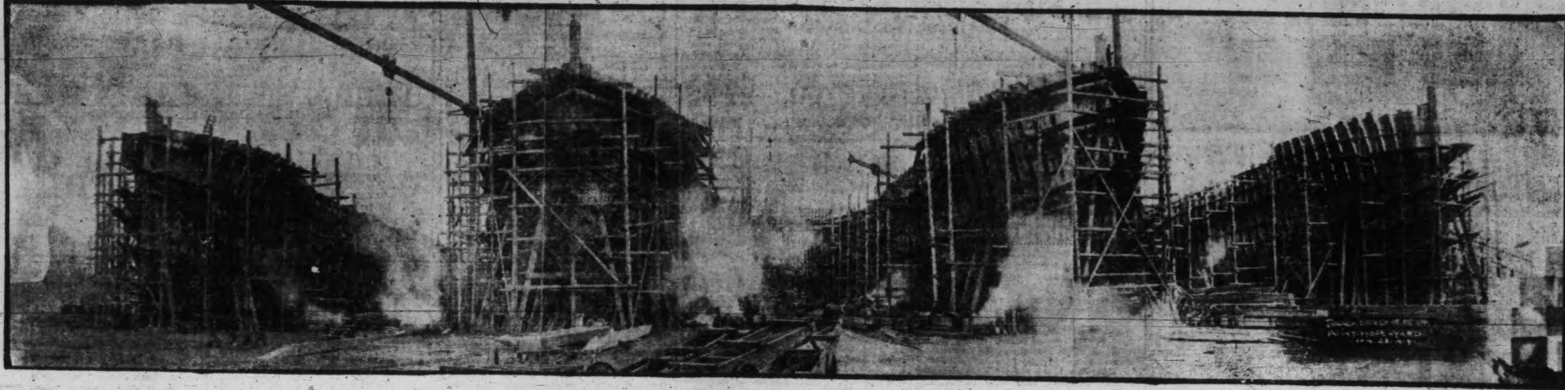
FOUNDATION COMPANY'S POINT HOPE SHIPYARD
