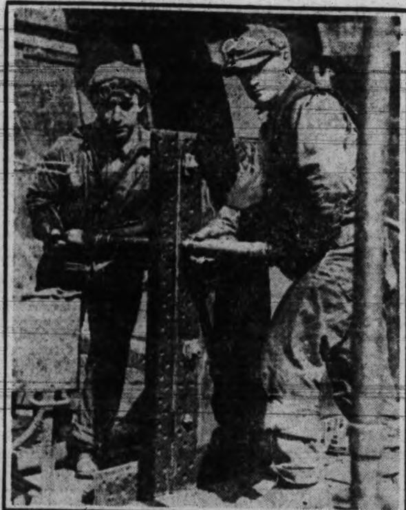
CHAMPION RIVET DRIVERS. —Robert Chambers (left) and William Heber. They are workmen of a shipbuilding plant at Quincy, Mass., and they hold the record for driving rivets. This team can drive rivets, seven-eighths of an inch thick at the rate of seventy a minute.
