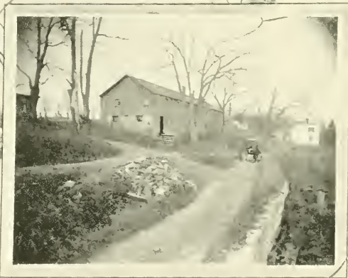
THE DRY HOUSE AND PORTION OF FOUNDATION OF THE FIRST CO-OPERATIVE CHEESE FACTORY IN THE WORLD.
