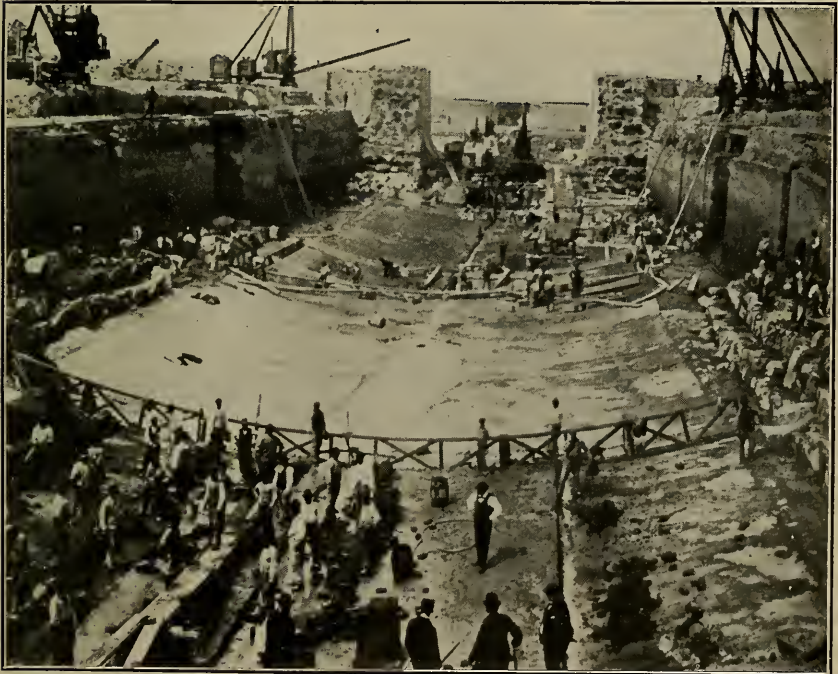
Here are shown the walls of the Pampean formation and alluvium still exposed after the concrete floor had been laid, with the sump and pumping machinery as in the view above.
