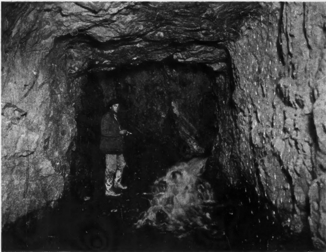
Good Hope Fluorspar Mine, Hardin County, Ill.—Water Entering 500-Ft. Level
