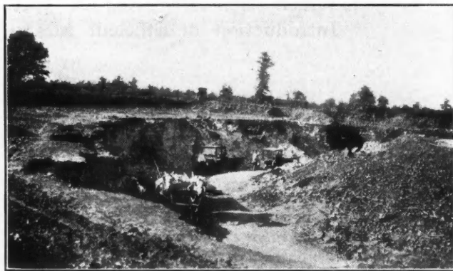
QUARRYING TRIPOLI NEAR SENECA, MO.
