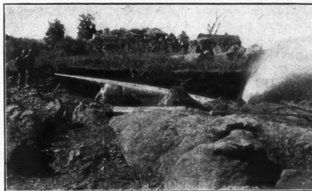
HYDRAULIC STRIPPING OF BEDFORD LIMESTONE, BEDFORD, IND.
