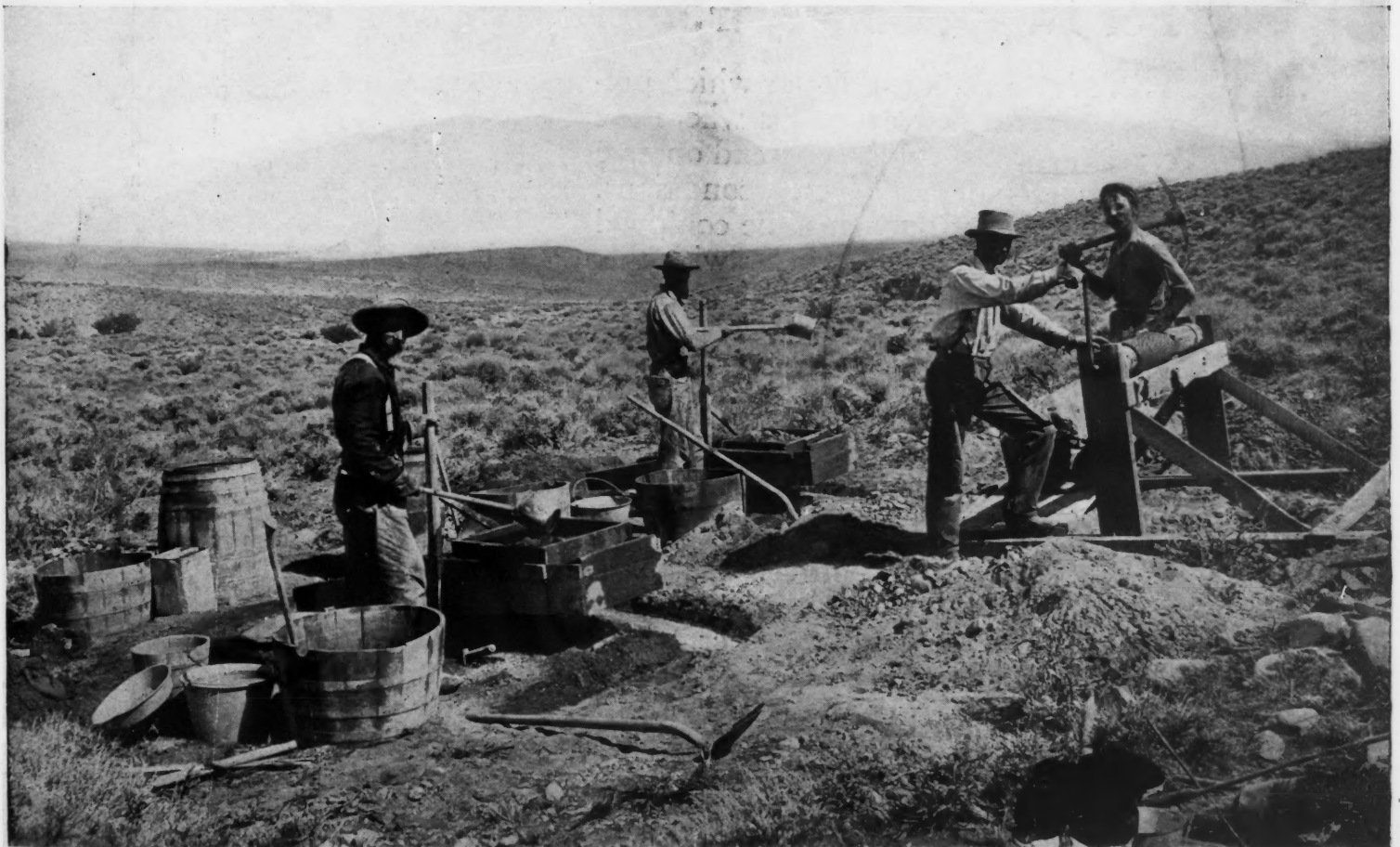
Test-Pitting Placer Dredging Ground in Nevada
