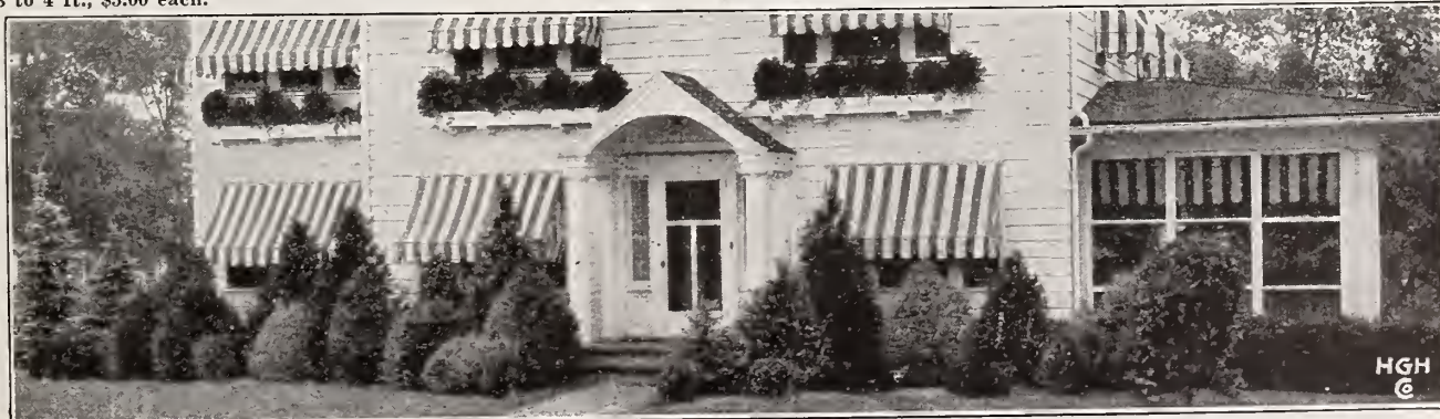
Very Effective Complete Foundation Planting and Window Box Arrangement, Using Coniferous Evergreens Entirely
