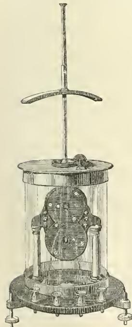
FIG. 5.—Thomson's double-coil astatic galvanometer.
