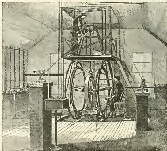
FIG. 2.—Large tangent galvanometer of Cornell University.
