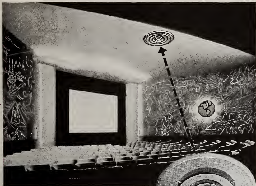
Trans-Lux Theatre, Modison Ave. at 85th St., New York City. Dwight D. Kimball, Engineer. Front orchestra view shows one large ceiling ANEMOSTAT which provides uniform and draftless air-distribution for mojour portion of the orchestra.
