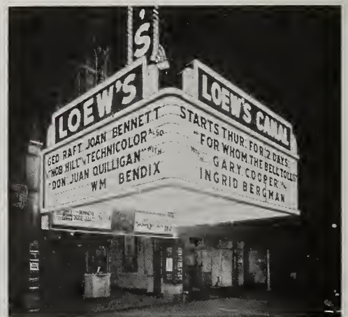
New installation of Adler removable panel attraction boards, with glass rounded corners, on Loew's Canal Street theatre, New York. Panels accommodate four lines of Adler silhouette letters.
