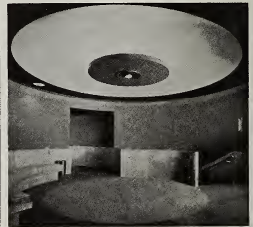
Hollywood Theatre, Sioux Falls, South Dakota. The circular ceiling Anemostat provided the motif for the interior decoration of this lobby. This striking design is typical of the varied effects obtainable with this device in association with lighting.
